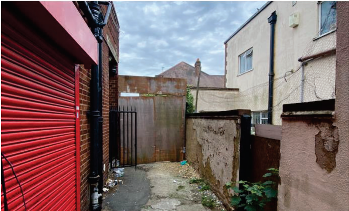
Figure 6: View from Alleyway between the site
