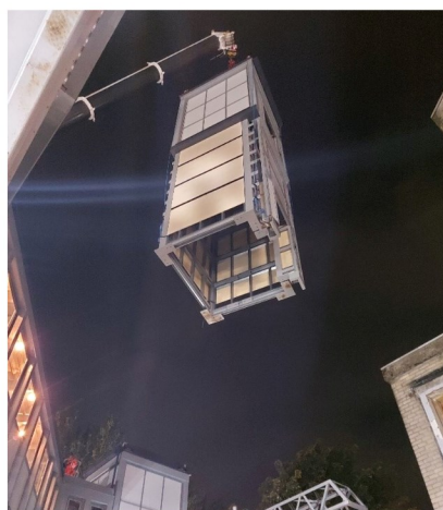
Hayes & Harlington—lift shaft craned in
