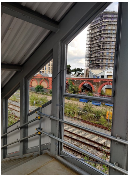
Southall—glazing frames installed
