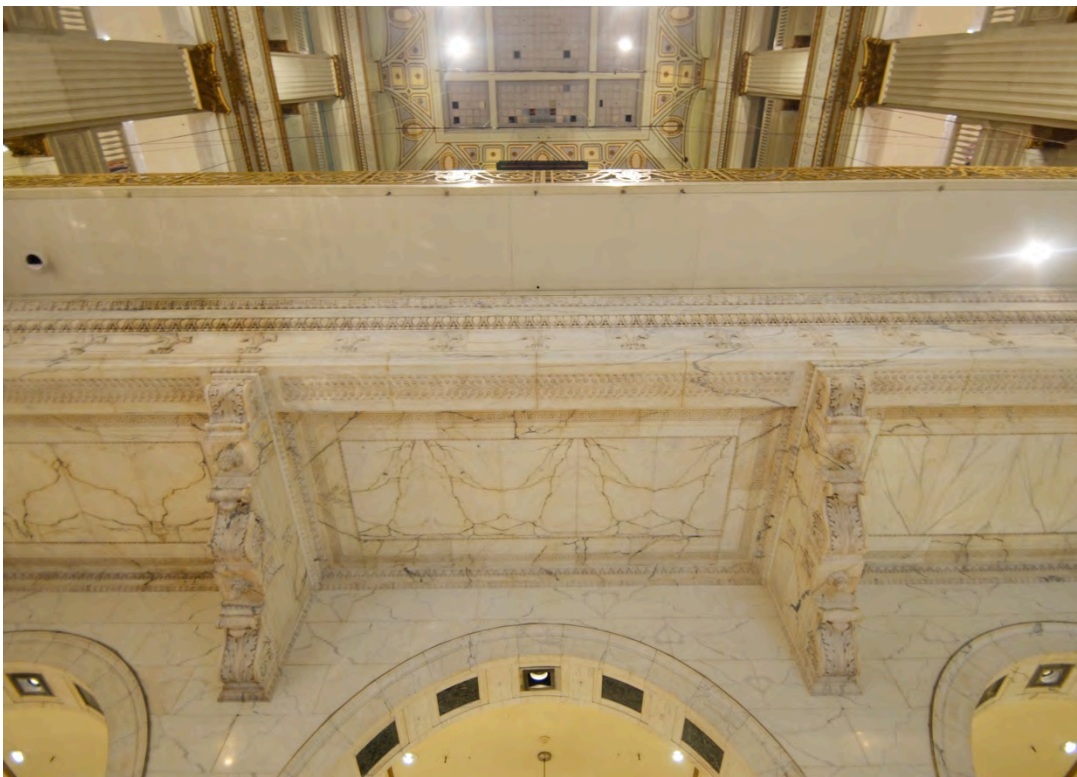
Figure 5: Balcony soffit and marble modillions beneath organ loft.
