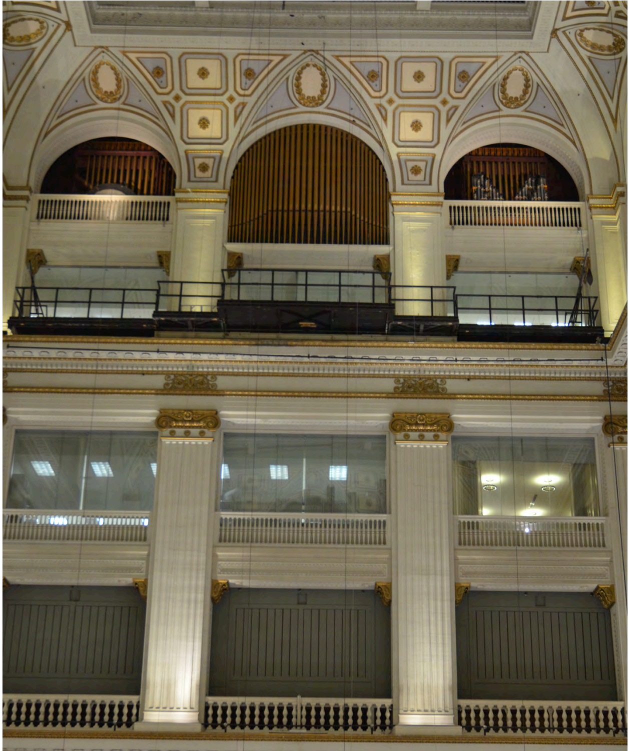
Figure 10: South gallery wall above organ loft, showing typical fifth-floor Ionic capitals, seventh-floor Doric capitals, groined coffered ceiling, and cast iron balustrades. Functional pipe divisions at seventh floor are contributing fixtures; glass partitions and contemporary scaffolding are non-contributing alterations.
