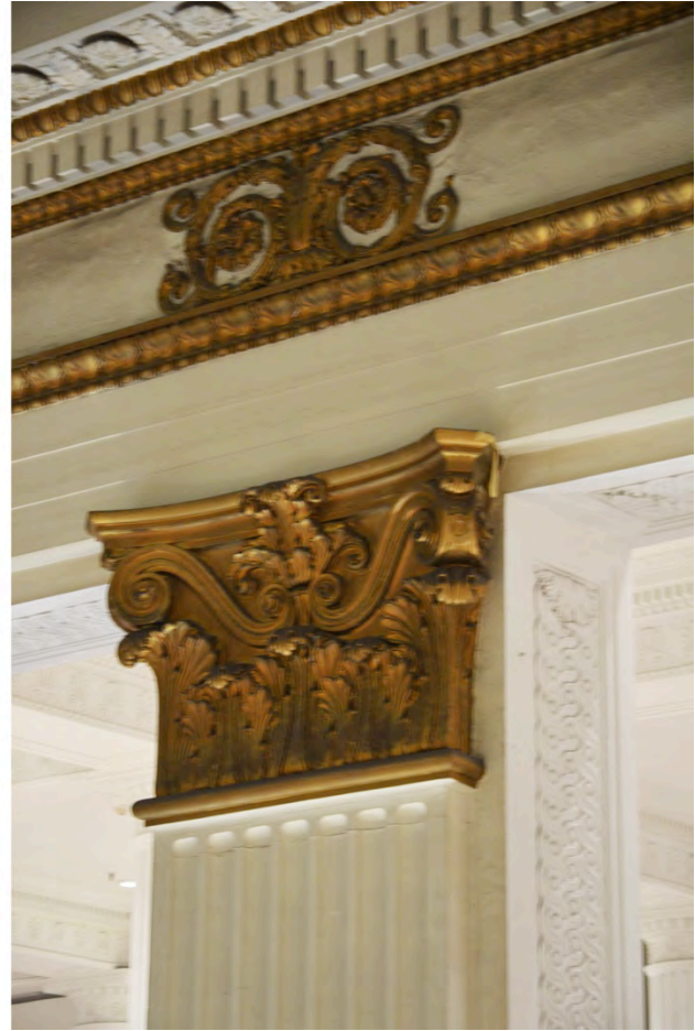
Figures 8-9: (L) Typical detail of second-floor colonnade, including ground-floor arcade cornice, spandrel panels between second and third floors, gilded modillion brackets, and cable-scrolled lateral column faces, all included in nominated area boundaries (R) Typical third-floor Corinthian capital detail and portion of projecting cornice.
