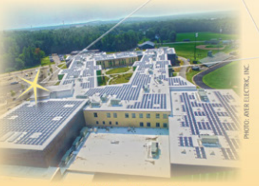
Dover High School, Dover, NH (New Hampshire's rooftop largest solar array)
