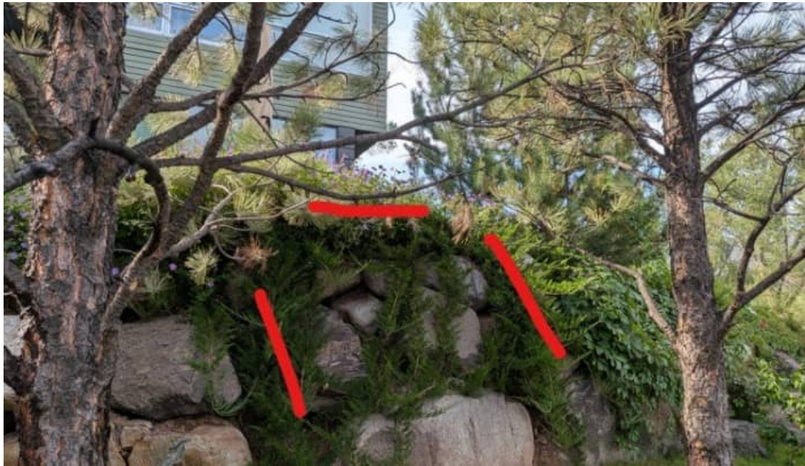
B5-5— remove ground junipers along wall
