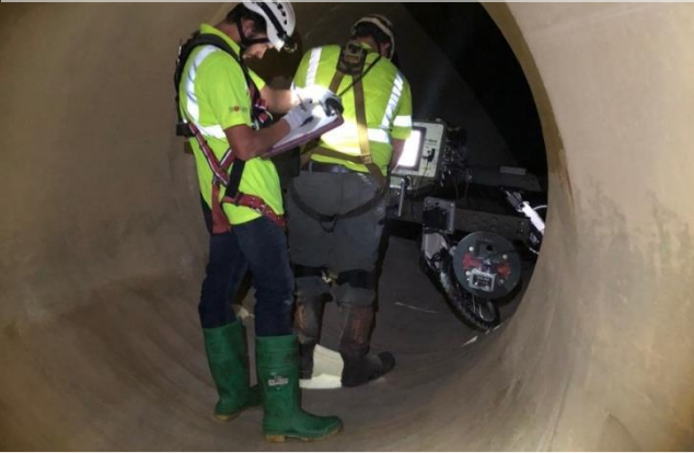
Rialto Pipeline PCCP Inspection
