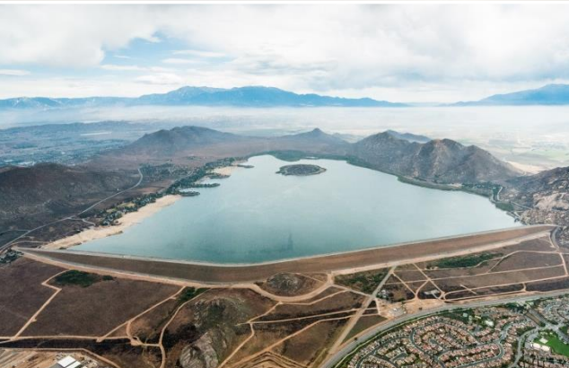
Lakeview/Perris Bypass Pipeline Relining
