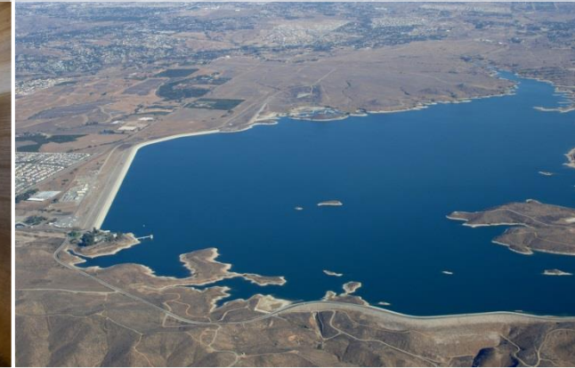
Lake Mathews Valves/Gates Maintenance
