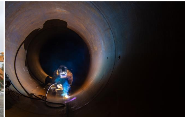
Allen-McColloch Pipeline PCCP Relining
