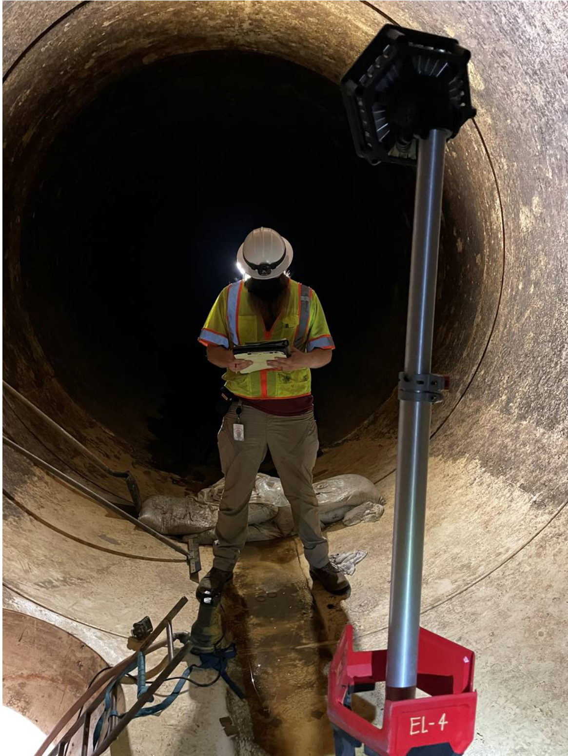
WSO's Scott Radel (Maintenance Engineering) records handheld laser measurements
