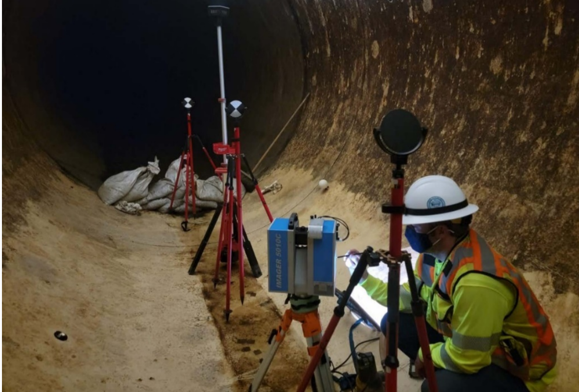
ESG's Matt Corcoran (Field Survey) preparing the 3D laser scanner to scan the Inland Feeder
