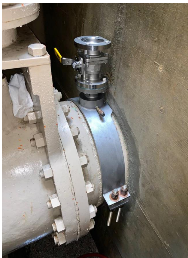
Fabricated saddle clamp for CB-01
