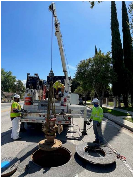
Carlos Marquez, Adam Guzman, and James Espinosa (C&D) removing a pipeline flange
