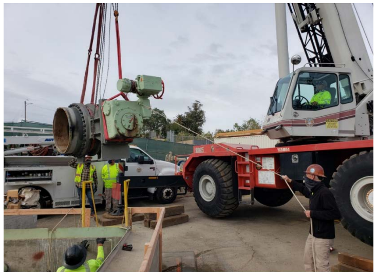
Dan Conover (CSU) mans the tag line while, Crane Operator David Jenkins (CSU) pulls out the old butterfly valve
