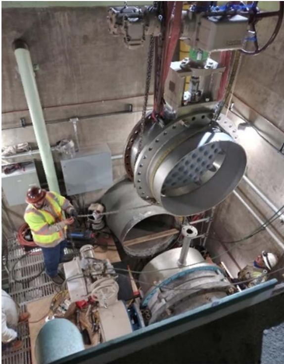
Paul Gonzalez installing the multi-orifice valve
