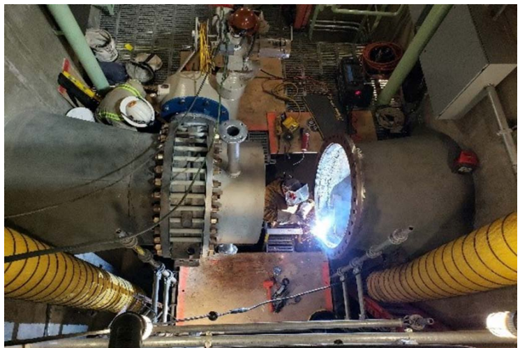
Luis Cortez welding a 42-inch flange
