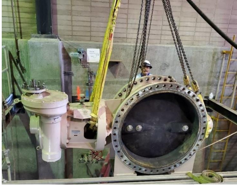
Juan Sandoval (C&D) removing a large valve to allow for pipe access at the Perris Pumpback facility
