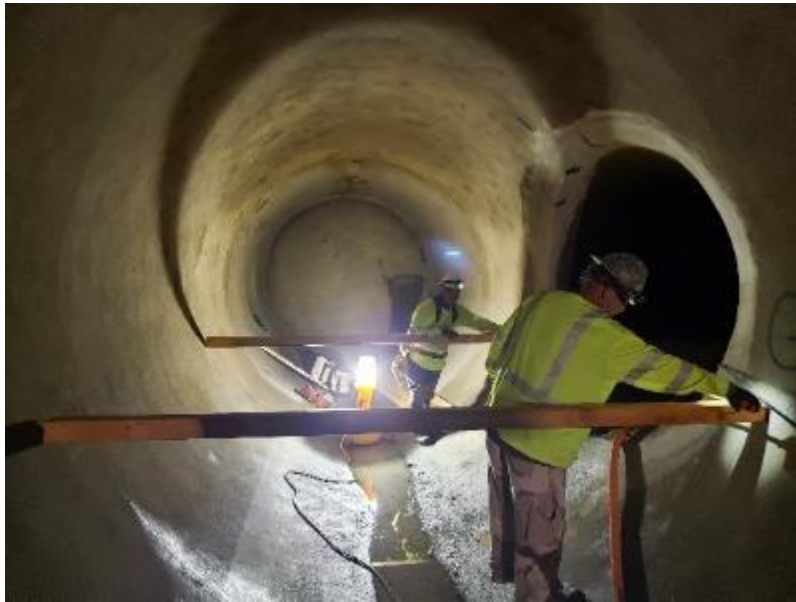
Chad Stone (right) and Daniel Finn (CSU) building scaffolding for pipeline coating removal at the Perris Pumpback facility
