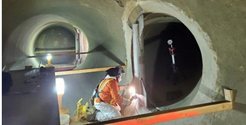
Dave Guerrero (C&D) welding prefabricated reinforcements into place at the Perris Pumpback facility
