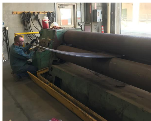
Welder/Fabricator Dave Paul (MSU) rolling top gusset for pipe reinforcement at the Perris
