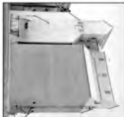
2. Metal-clad elevator with metal-clad annex.
