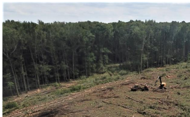
Figure 3. Shovel logging with cut trees to construct a temporary skid trail. Image credit: Patrick Hiesl, Clemson University.
