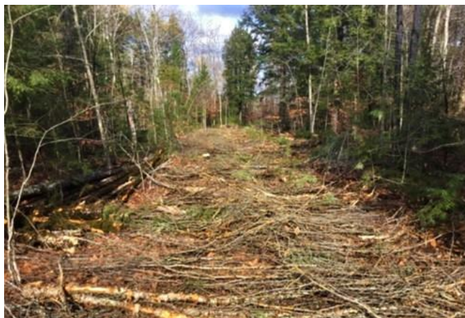
Figure 4. Application of slash in the forest skid trail. Image credit: Courtesy of Maine Forest Service - Forest Policy and Management.
