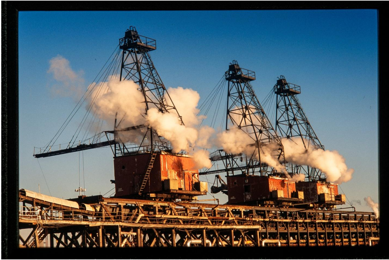
A shore-side boiler provided steam to the three Sprague Energy cranes. Peggy McKenna Collection, LB2915.11.5878.17.
