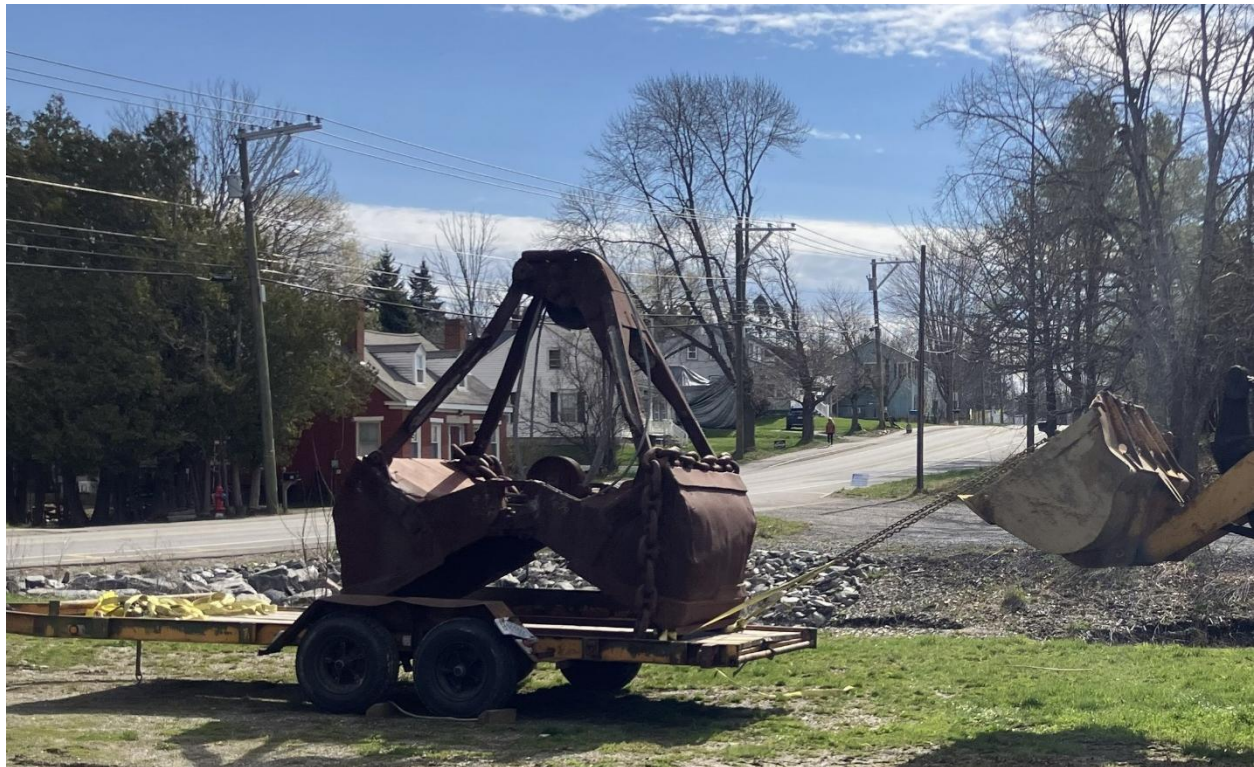
The grab bucket arrives in Searsport, where the town crew prepares to unload it. It holds 2 ½ cubic yards of material. Image courtesy of Cipperly Good.
