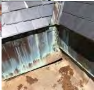
Existing flashing
