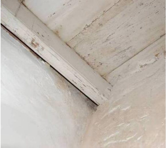
Limewashed wood ceiling and plaster walls at the 1730 Newbold-White House in Perquimans Co.
