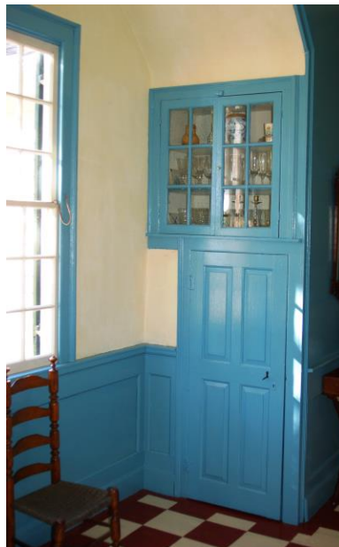
Tinted lime paint on sheetrock wall and ceiling (left) and plaster (right) in this 19 th century Martin Co. Farmhouse.
