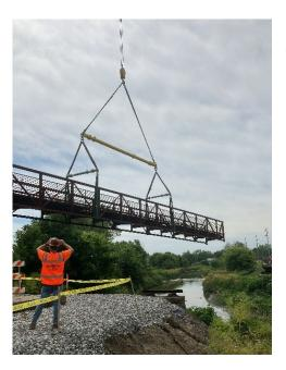
The existing pedestrian bridge across the Little Calumet River was removed, salvaged for reinstallation, and is currently stored on-site.
