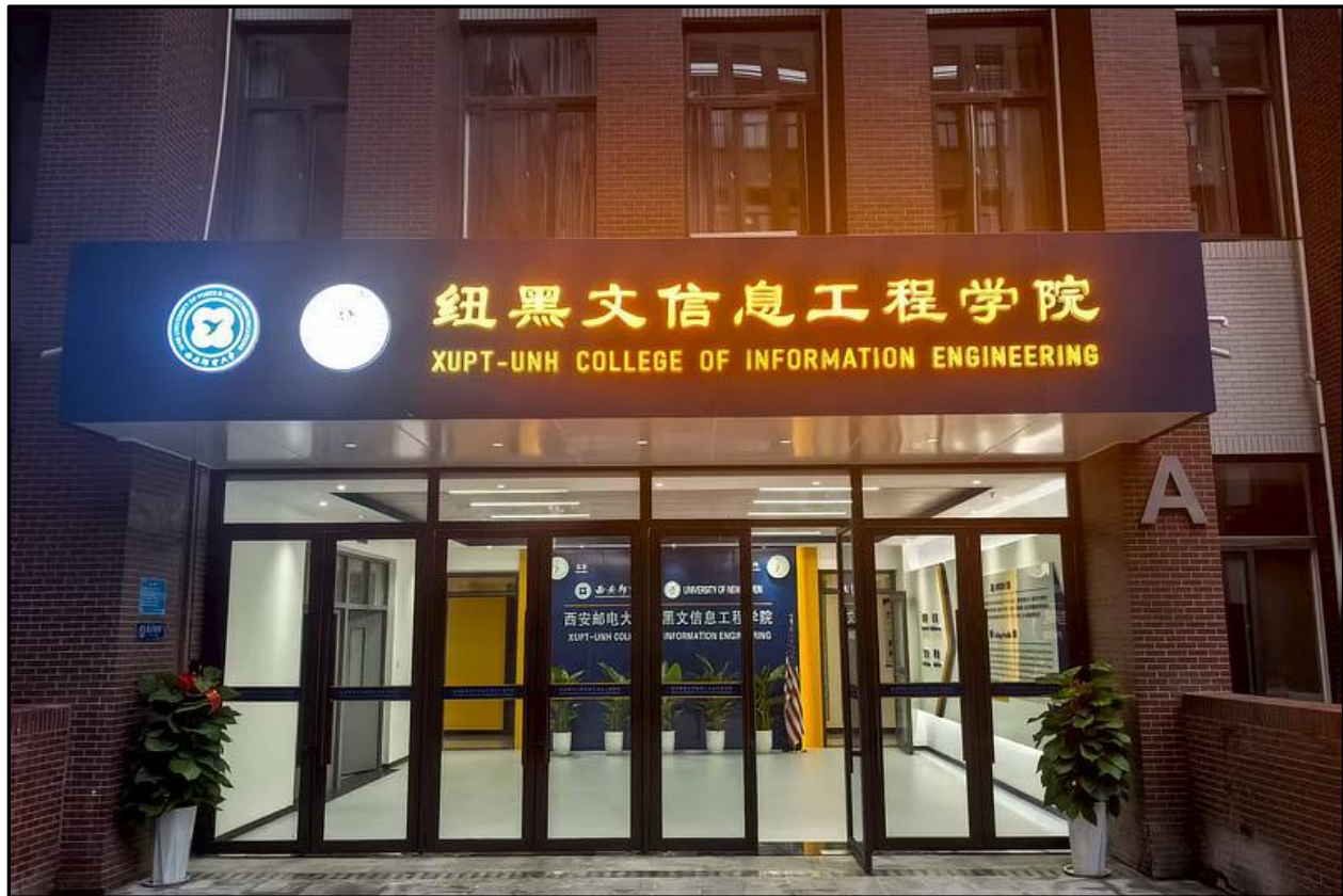
Figure 1: XUPT-UNH College of Information Engineering Building at Xi'an, Shaanxi Province, China
