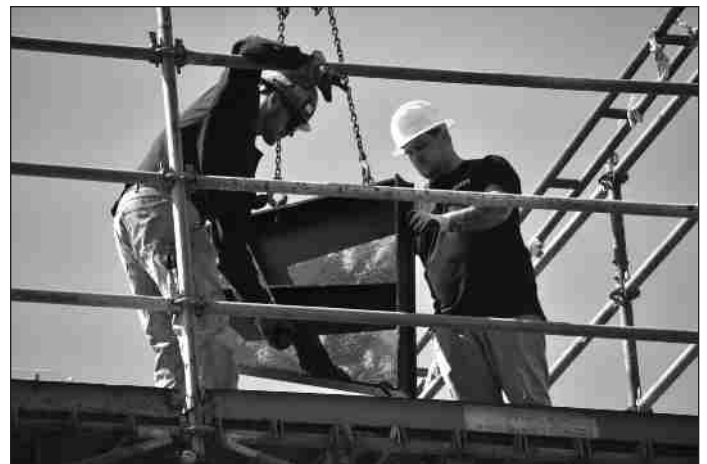
At least 100 new castings were created for renovating the lighthouse tower. Nick Bliler and Ryan Strack are about to uncouple from the crane another exterior gallery plate. Each weighs roughly 180 pounds and there are 16 of them. Photo by Kim Fahlen.
