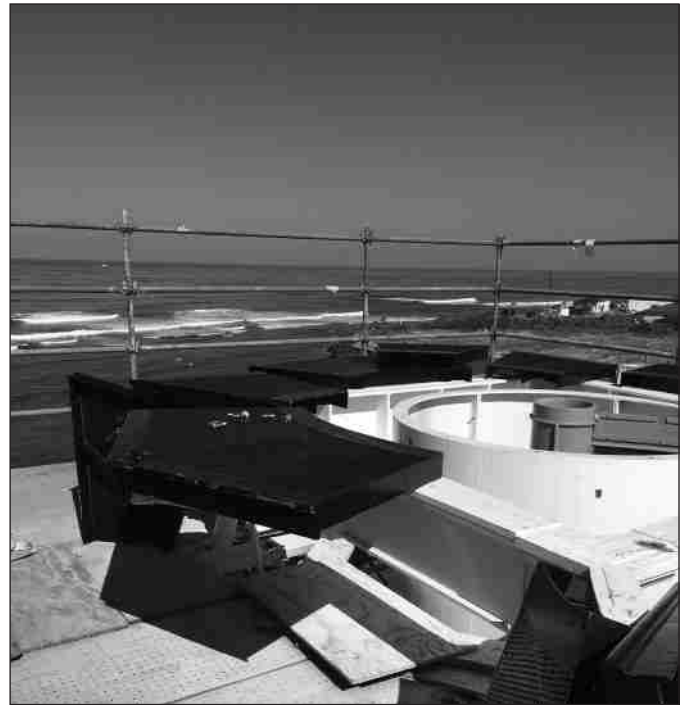
Above left: Easing into its mate underneath is the first recast cylinder wall plate. Note stairs on right, which soon will be encircled and out of view from outside after five companion wall plates are bolted together. Courtesy of Kim Fahlen
