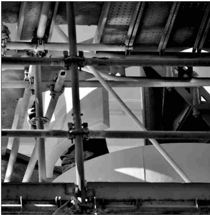
Above left: Easing into its mate underneath is the first recast cylinder wall plate. Note stairs on right, which soon will be encircled and out of view from outside after five companion wall plates are bolted together. Courtesy of Kim Fahlen
