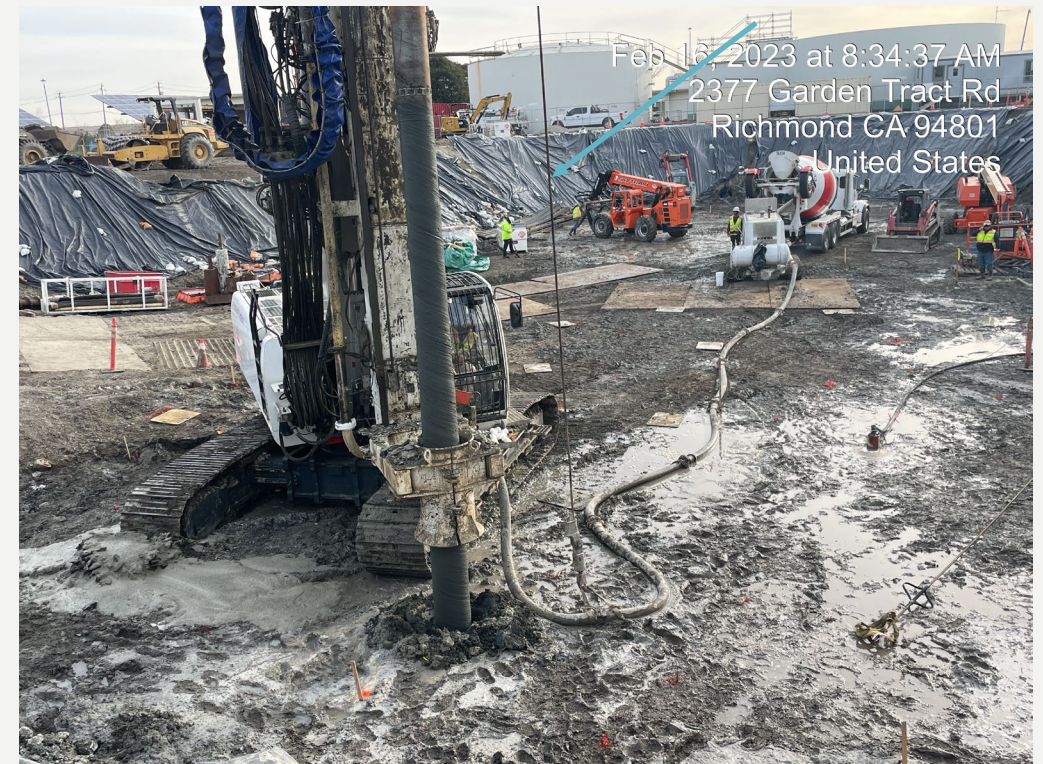
Drilling and placing grout for DDC for digester foundation
