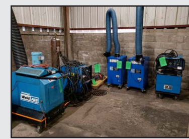
MULTIPLE WELDERS AND FUME EXTRACTION
