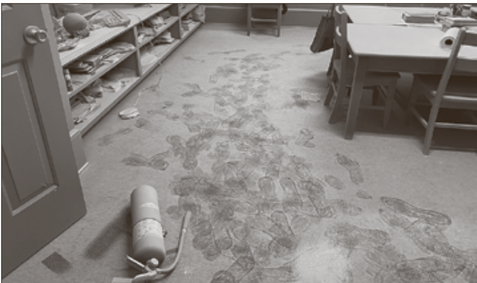
Fire extinguisher dust caused the worst damage, such as to this children's classroom.
