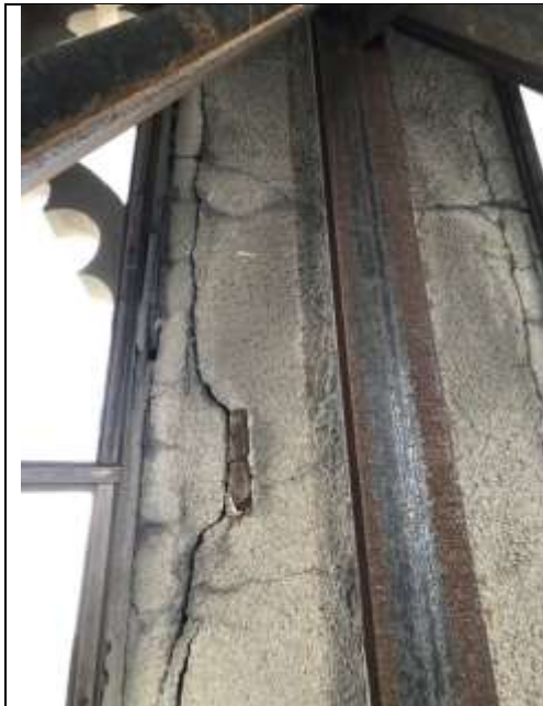
Failing inside of tower
