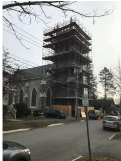
Scaffolding during tower removal
