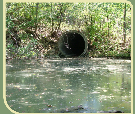
Stormwater outfall
