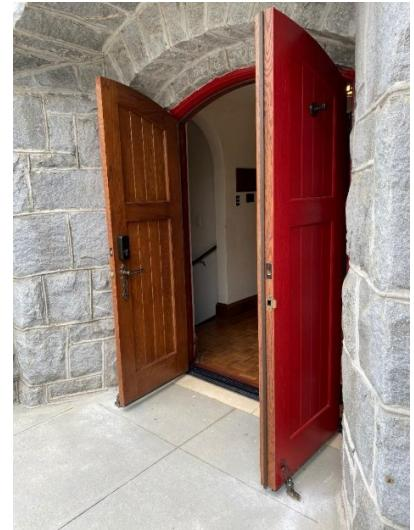
These doors are 2 inch white oak, which should stand sturdy for at least 75 years! The detail work is carved on the surface, so panels won't shrink apart in years to come. The non-handle door uses sliding surface locks on top and bottom, which are much more durable than in-door floor and ceiling locks.
