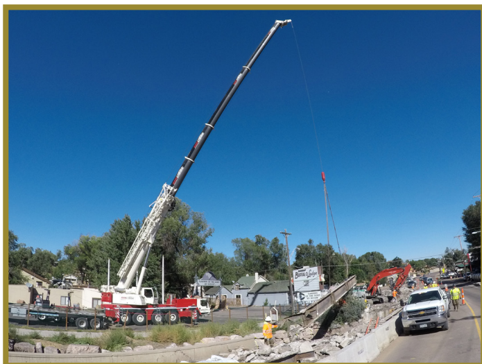
Removing steel girder from the bridge over Fountain Creek
