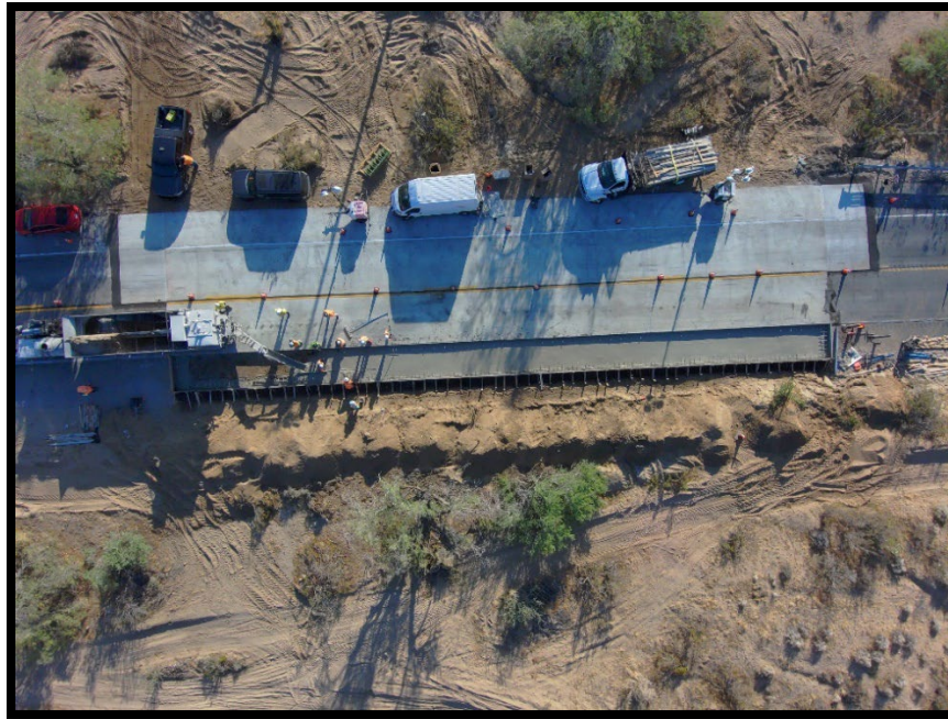
Figure 1 June 2025 Concrete Pour
