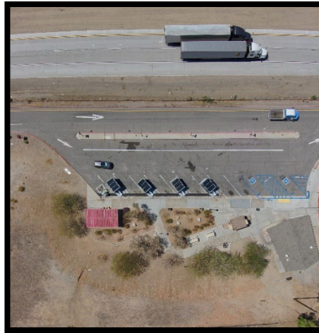
Figure 2 top-down drone aerial photo Cactus City SRRA
