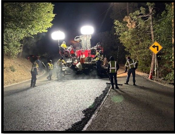
Figure 1 Nightwork Paving
