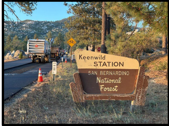
Figure 2 Paving at Keenwild Station
