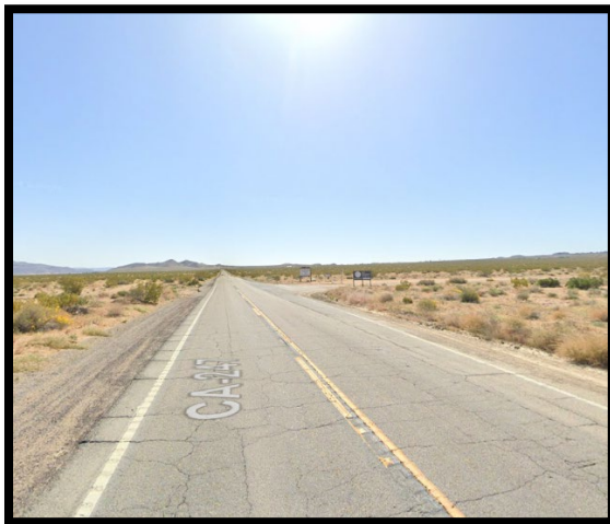
Figure 2 SR-247 Before Road Improvement Near Larrea Rd Photo
