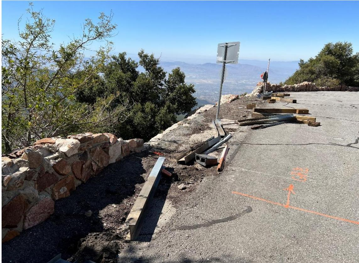
Location 3 after (below): excavation complete – will install soil nails, concrete pad.
