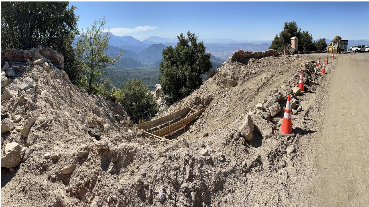
Location 1 before (below): removal of guardrail and starting on historical wall removal
