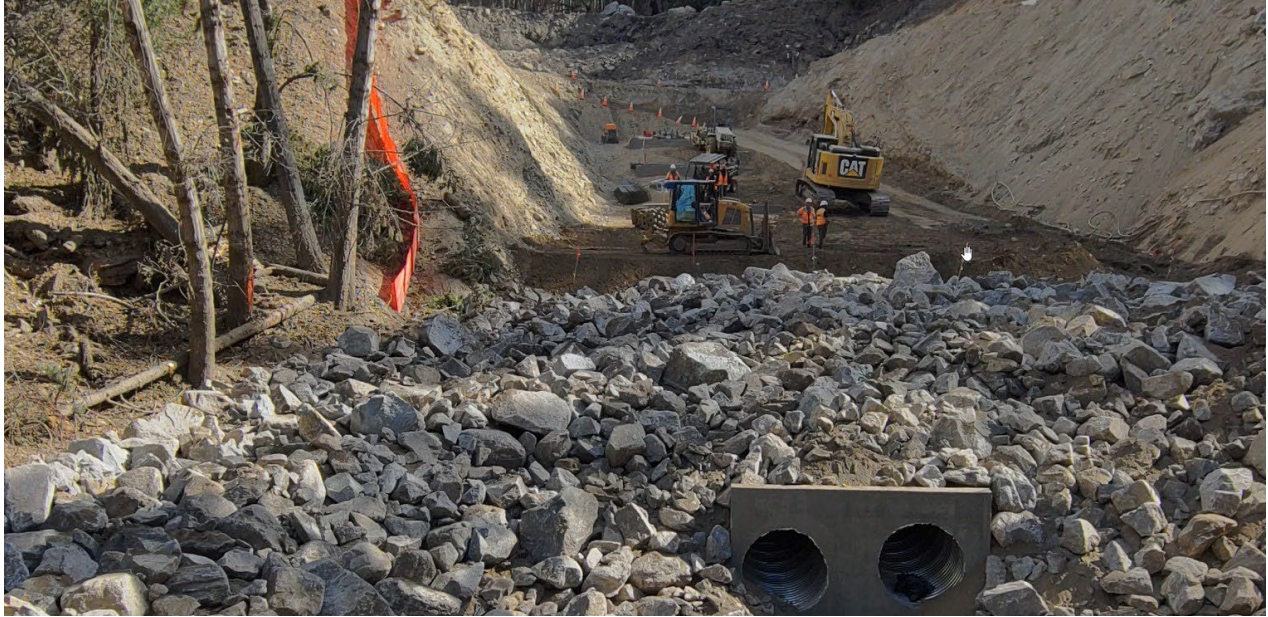
Postmile 23.90 Culvert Installation at Washout Location
