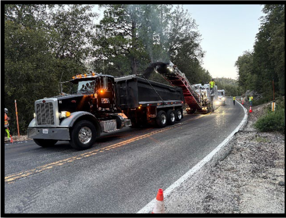
Figure 2 Grind and Pave operations
