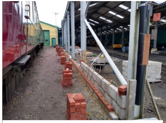
The photo shows the beginnings of the dwarf wall on the western side of the maintenance road.
