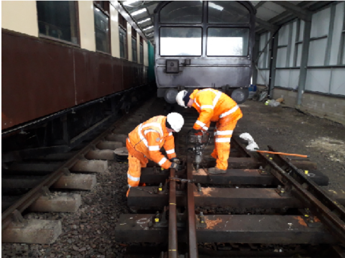
Building the switch blade section of the A road points.
