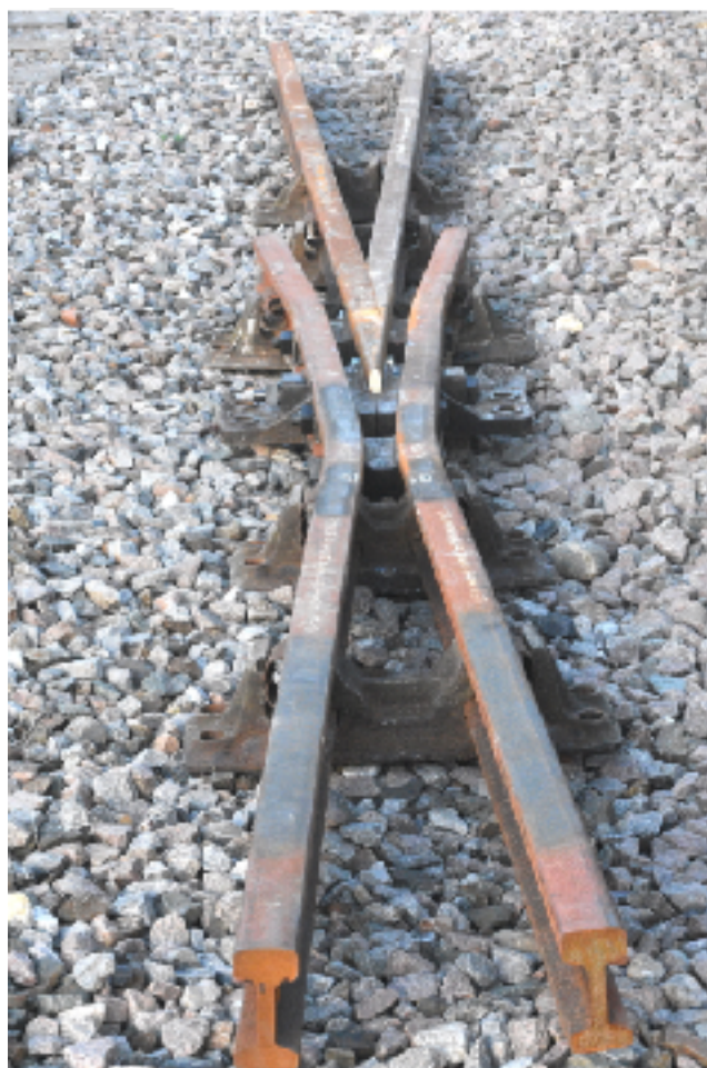
New A road crossing nose freshly assembled.
