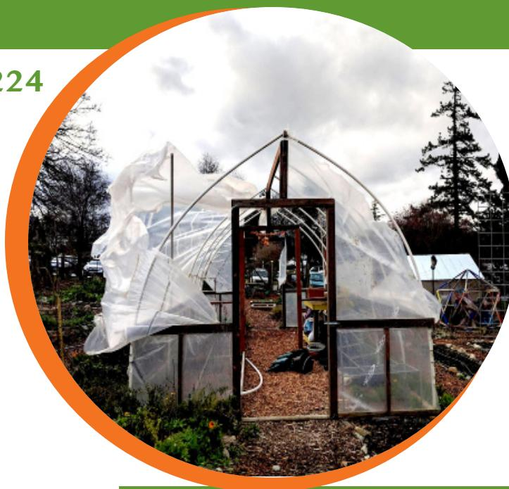
Winter winds deconstructed our temporary greenhouse, a 12'x24' gothic arch structure of recycled plastic that lasted 2 years.
