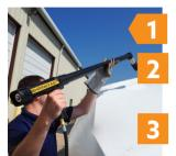
Completely shrink the cover before installing vents.
