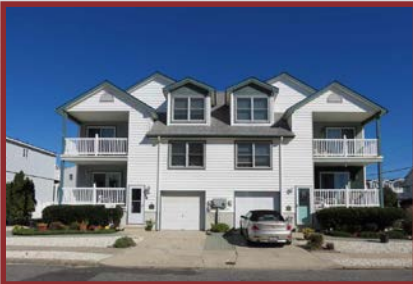
JUST REDUCED! NEVER BEEN RENTED AND ONLY ONE OWNER. (7212 Landis Ave West Unit) Five-bedroom, three bath and one-half bath multi-level townhouse. $765,000
