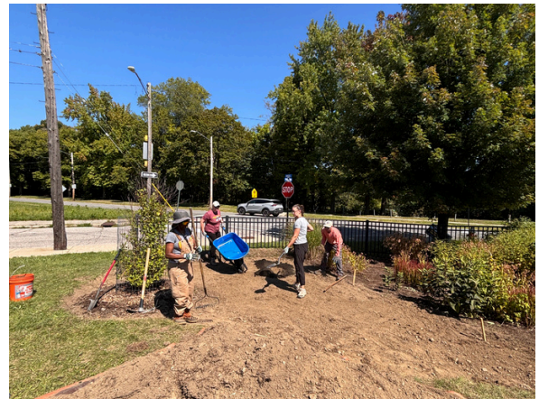
Volunteer Master Rain Gardeners remove soil for a rain garden at Wilson Elementary School in Cleveland, Ohio.
