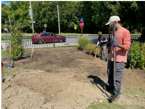
Volunteer Master Rain Gardeners amend soil for a rain garden at Wilson Elementary School in Cleveland, Ohio.
