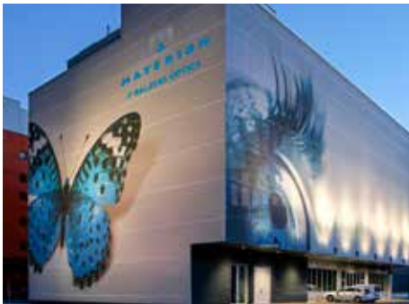
Production Balzers/Principality of Liechtenstein
