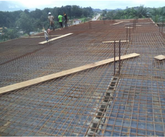
Construction of slab for second story of Jasper Grant UMS annex, Pleebo, Maryland County.
