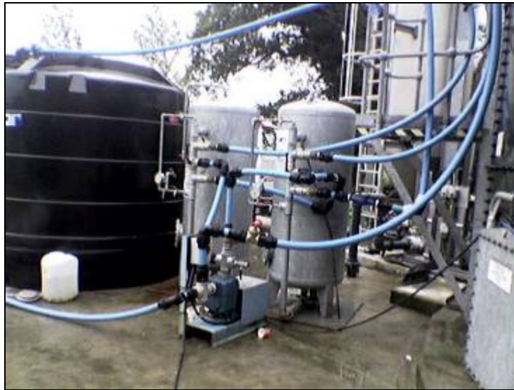
Figure 4. Two-stage filtration system
