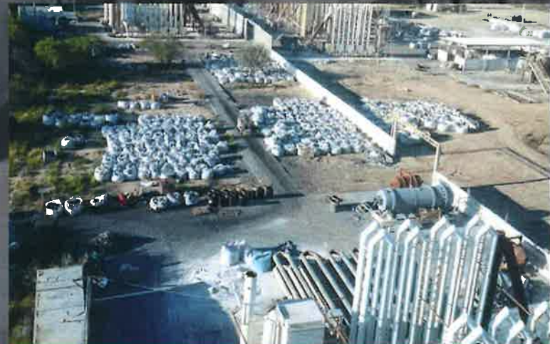
MADERO SMELTER PLANT - COAHUILA, MEXICO NOTE: SMELTER CAPACITY OF 200 TONS PER MONTH OR 7 TONS PER DAY
