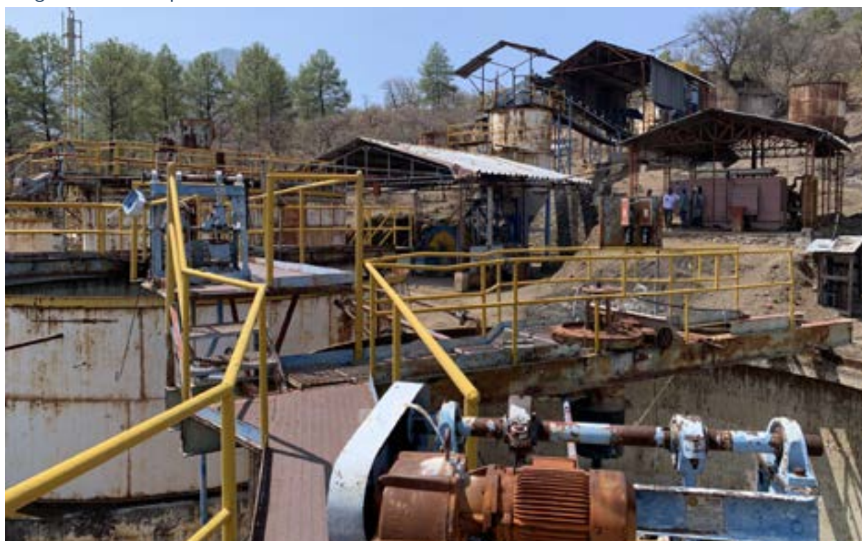
Image 3: El Potrero plant from below
