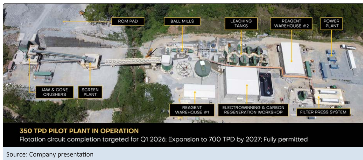
Figure 9: Tuvatu Gold Project — 350 TPD pilot plant
