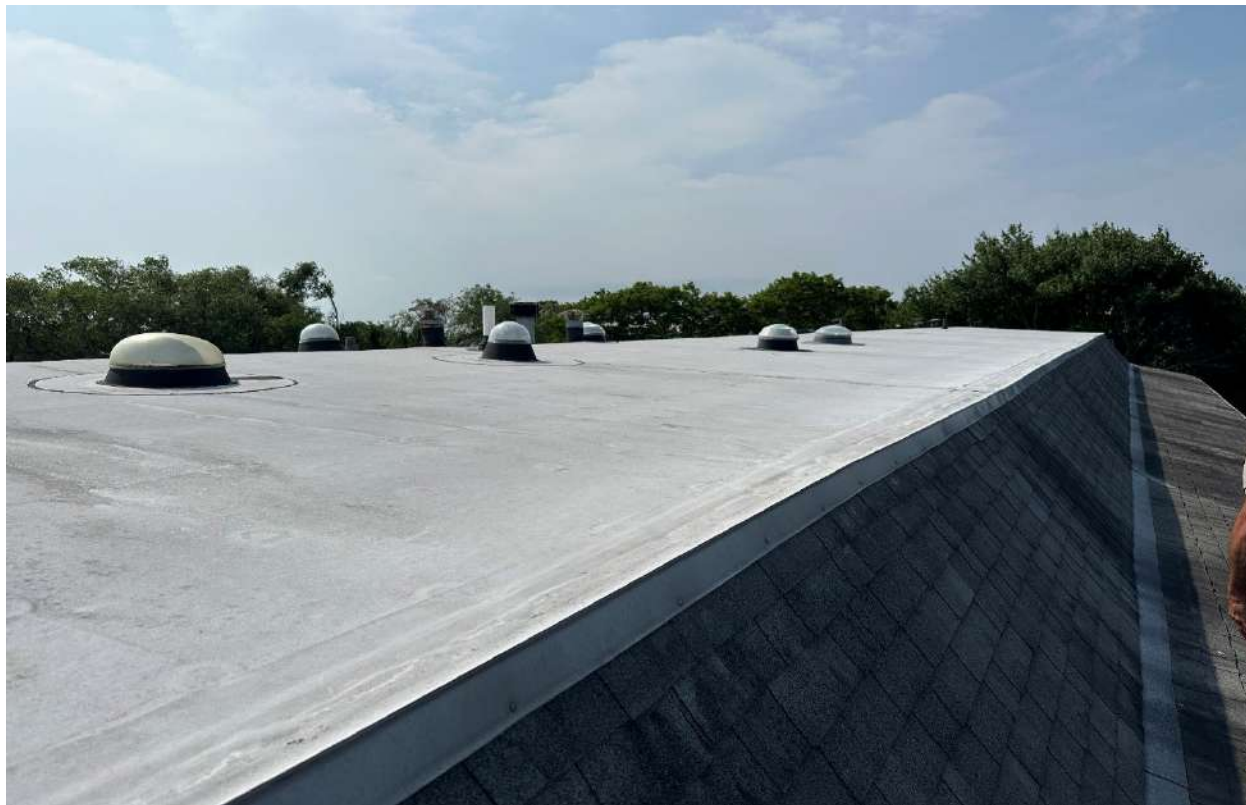
P-54 Solar Tube Skylight Missing Flashing
