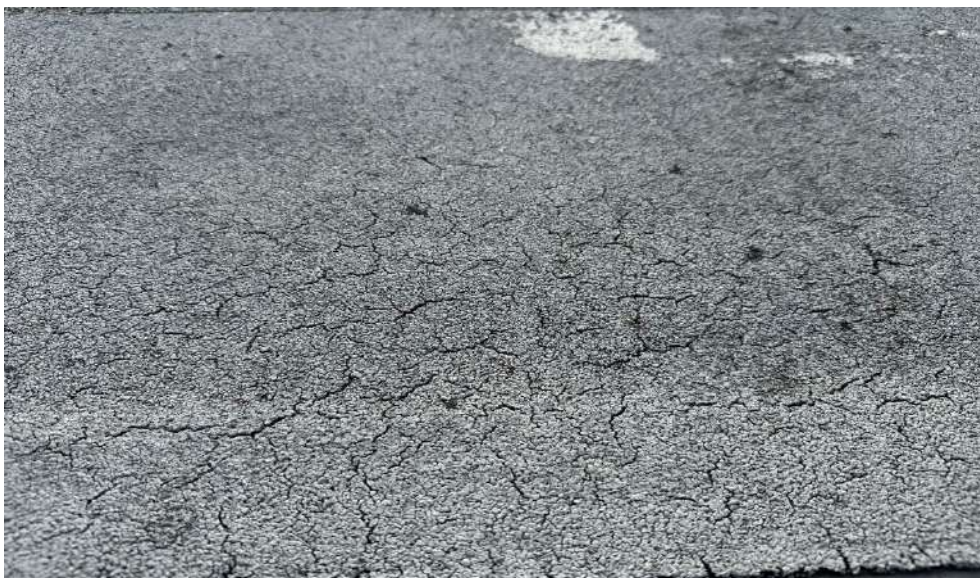
P-20 Alligatoring in Membrane
