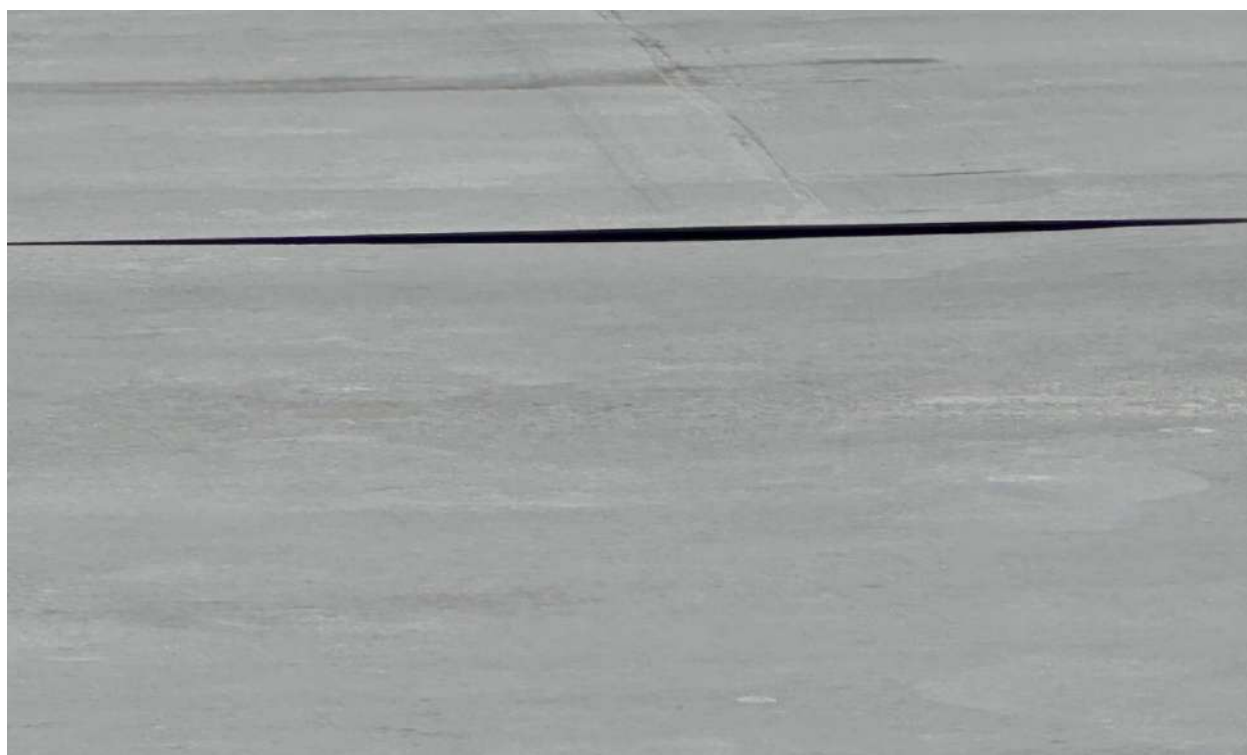
P-58 Fish mouth in TPO Membrane
