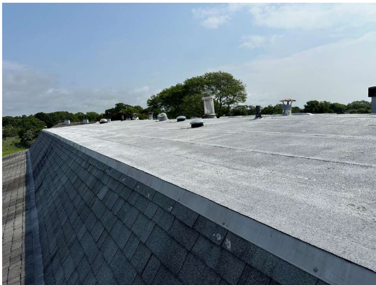
P-67 Overall of Roof
