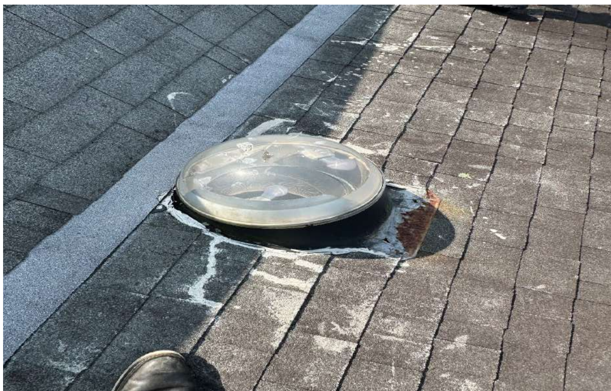
P-86 Sealant Added At Solar Tube Flashing
