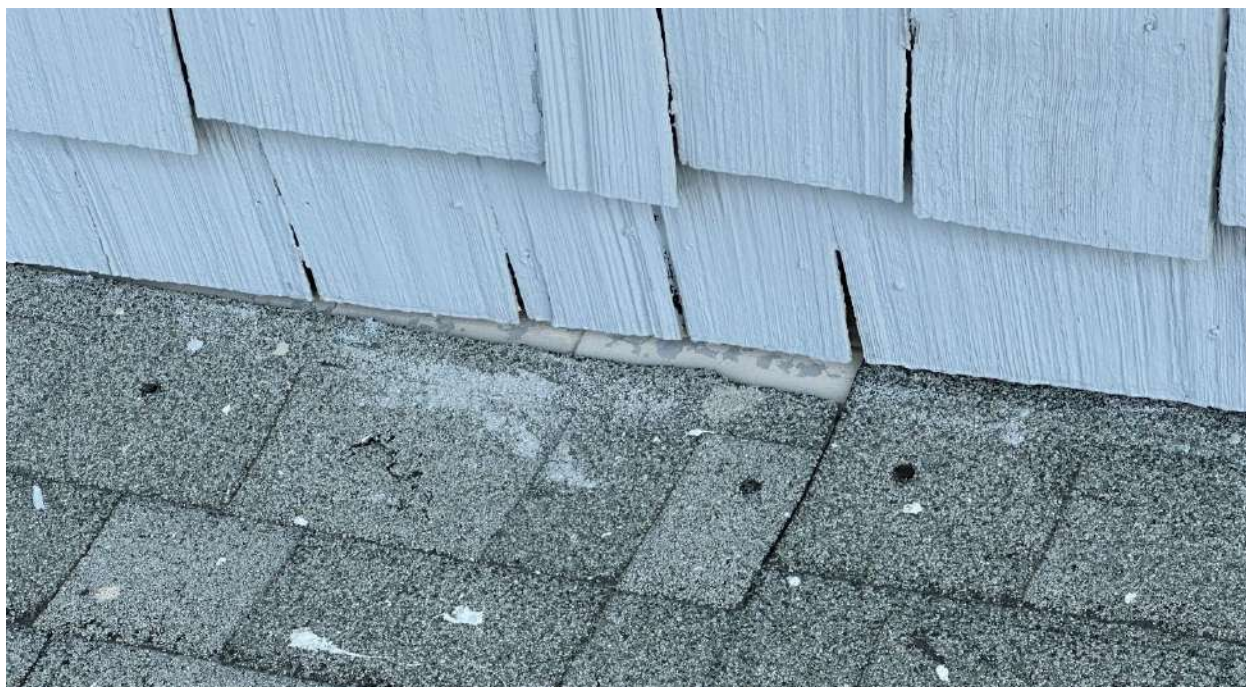
P-50 Loose Shingle and Exposed Fasteners
