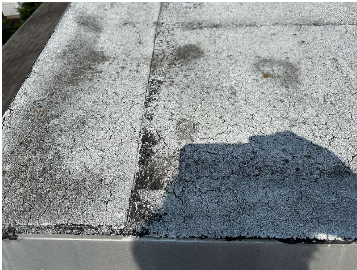
P-69 Alligatoring in Membrane
