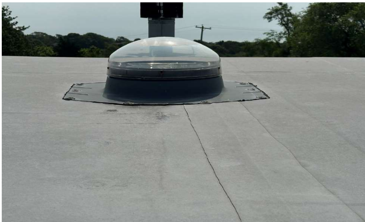
P-54 Solar Tube Skylight Missing Flashing
