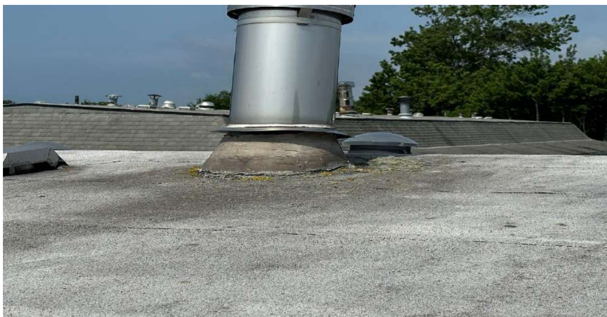
P-70 Chimney Penetration
