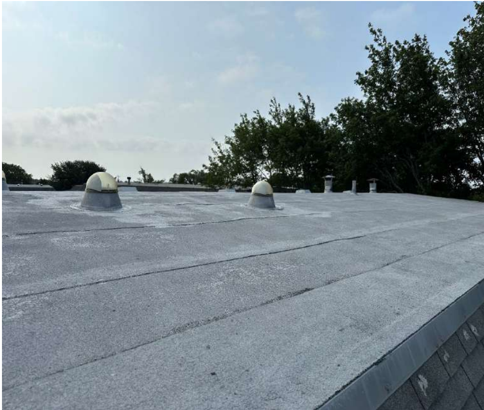
P-20 Alligatoring in Membrane
