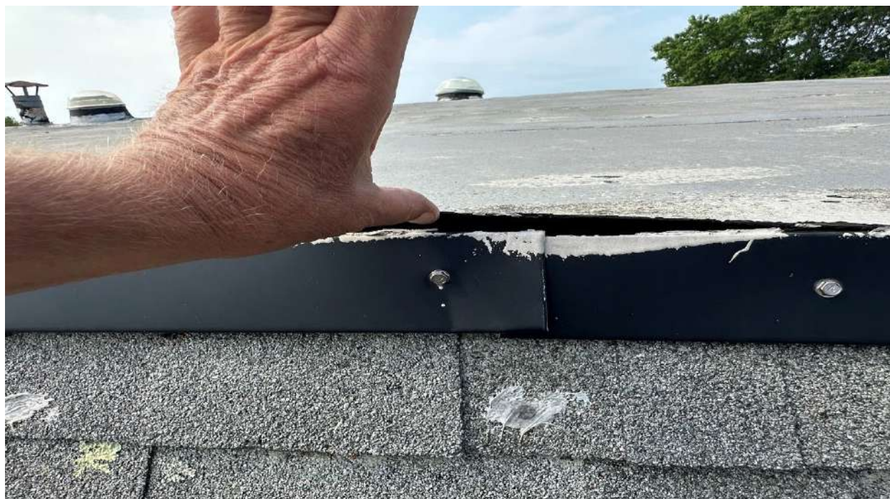
P-37 Opening in Membrane at Edge Metal
