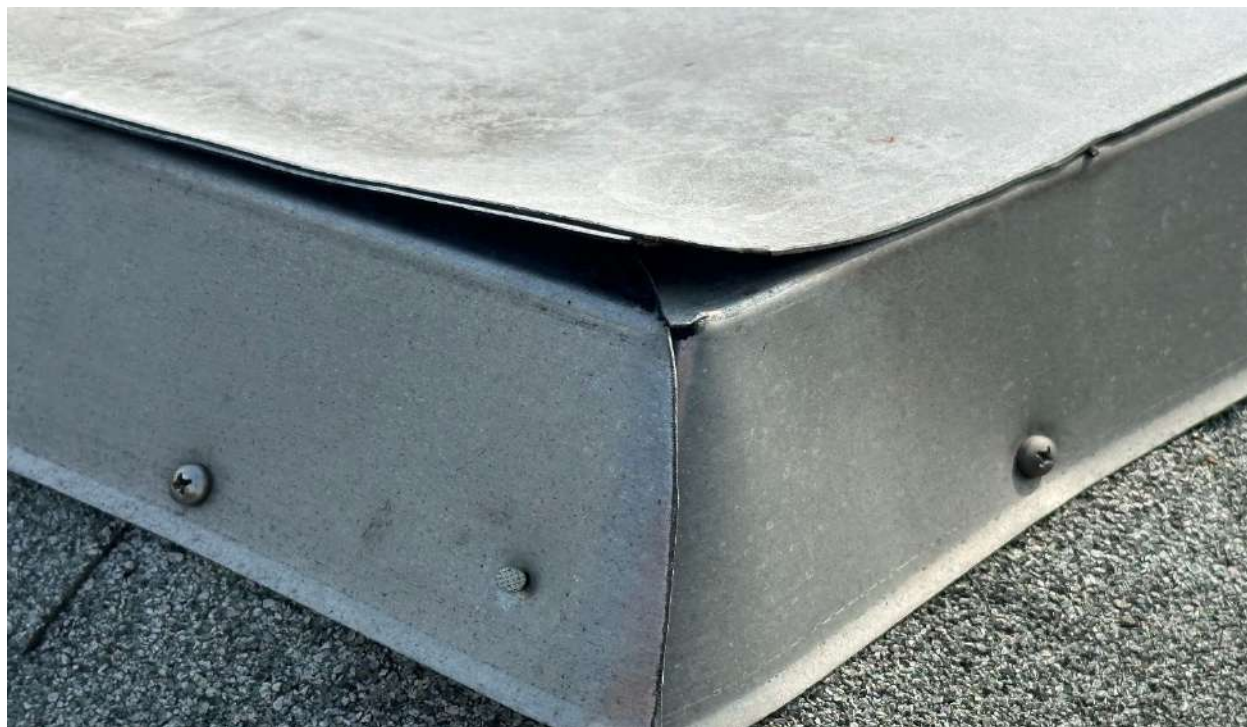
P-58 Fish mouth in TPO Membrane
