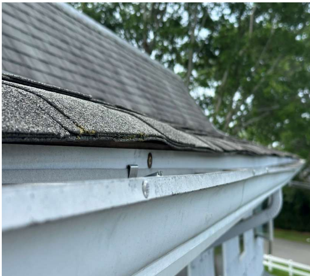
P-18 Prior Replaced Shingles
