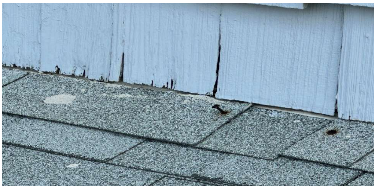
P-76 Rusted Exposed Shingle Fastener
