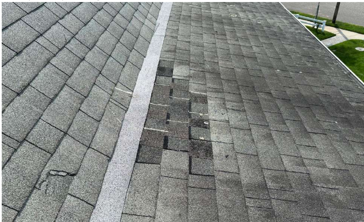
P-59 Replaced Asphalt Shingle
