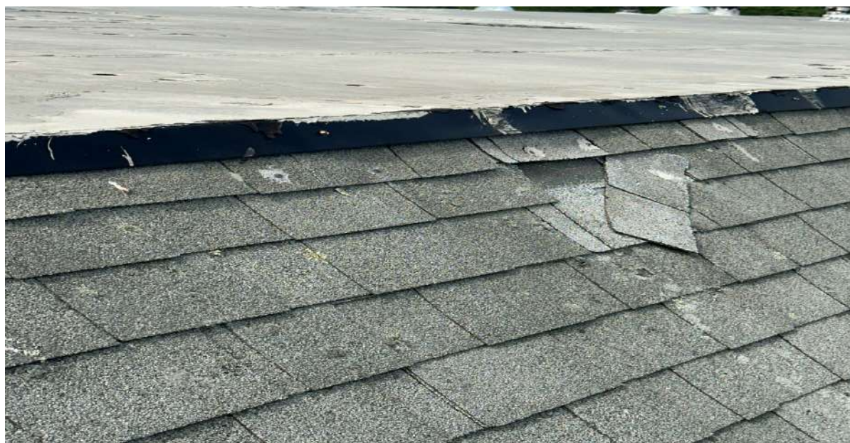
P-43 Delaminating Shingle
