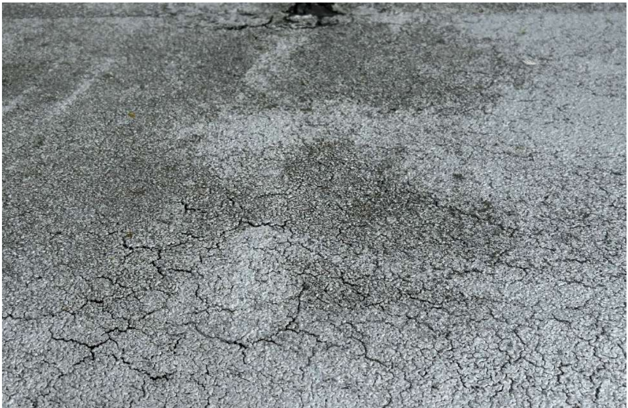
P-7 Alligatoring of Membrane
