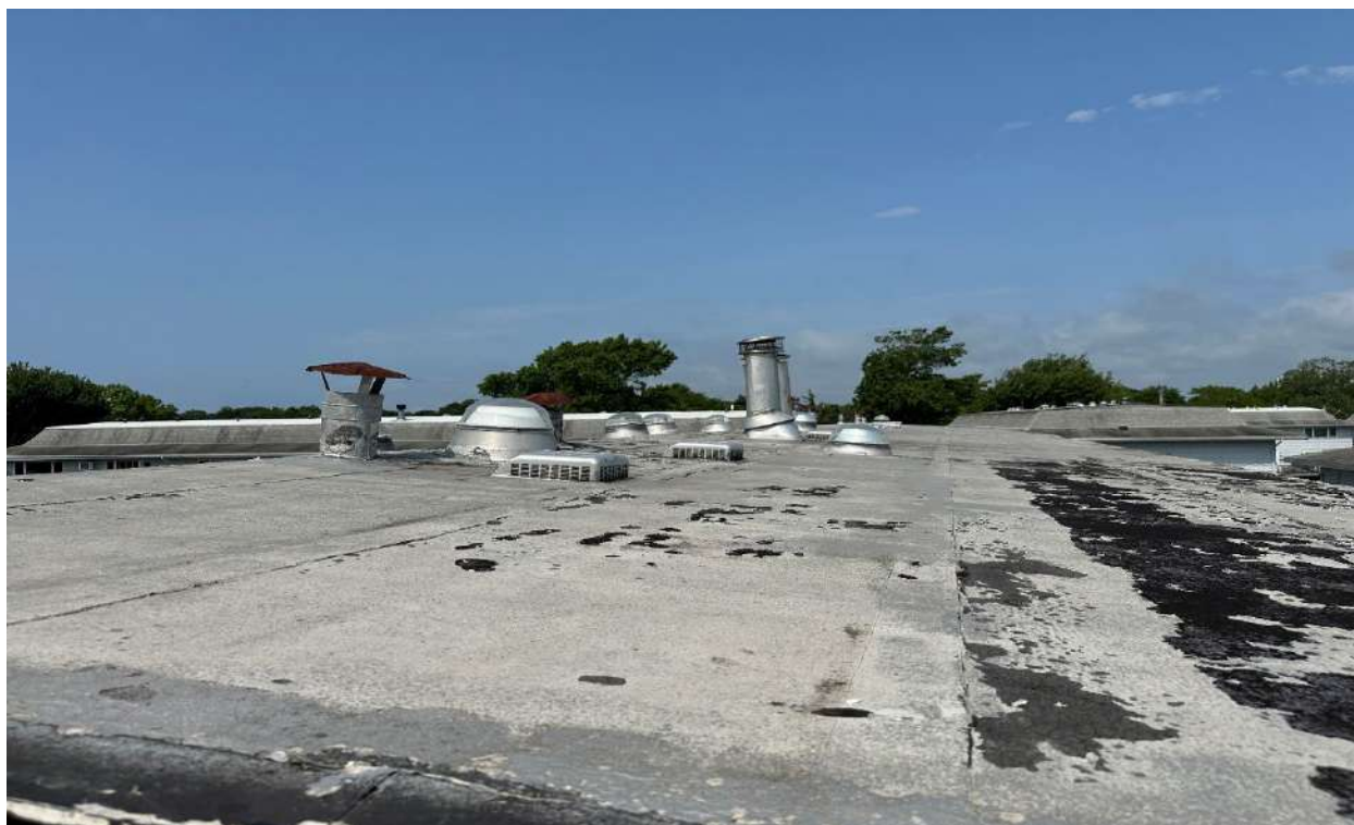
P-84 Overall Of Roof
