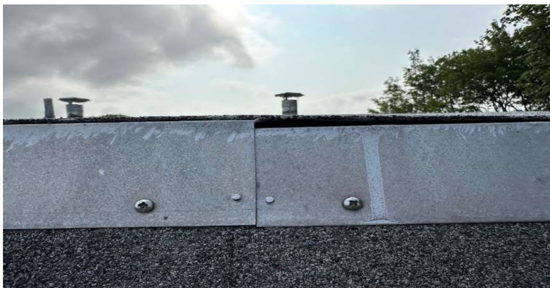
P-26 Gap at Fascia and Shingle Exposing Sheathing
