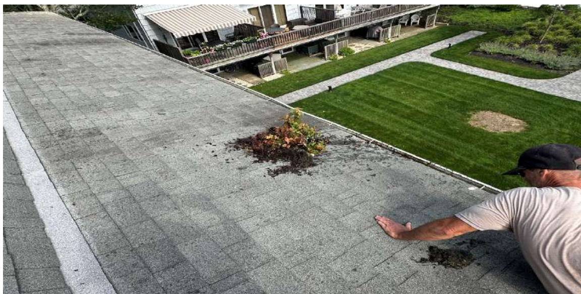
P-47 Leaf Matter in Gutter
