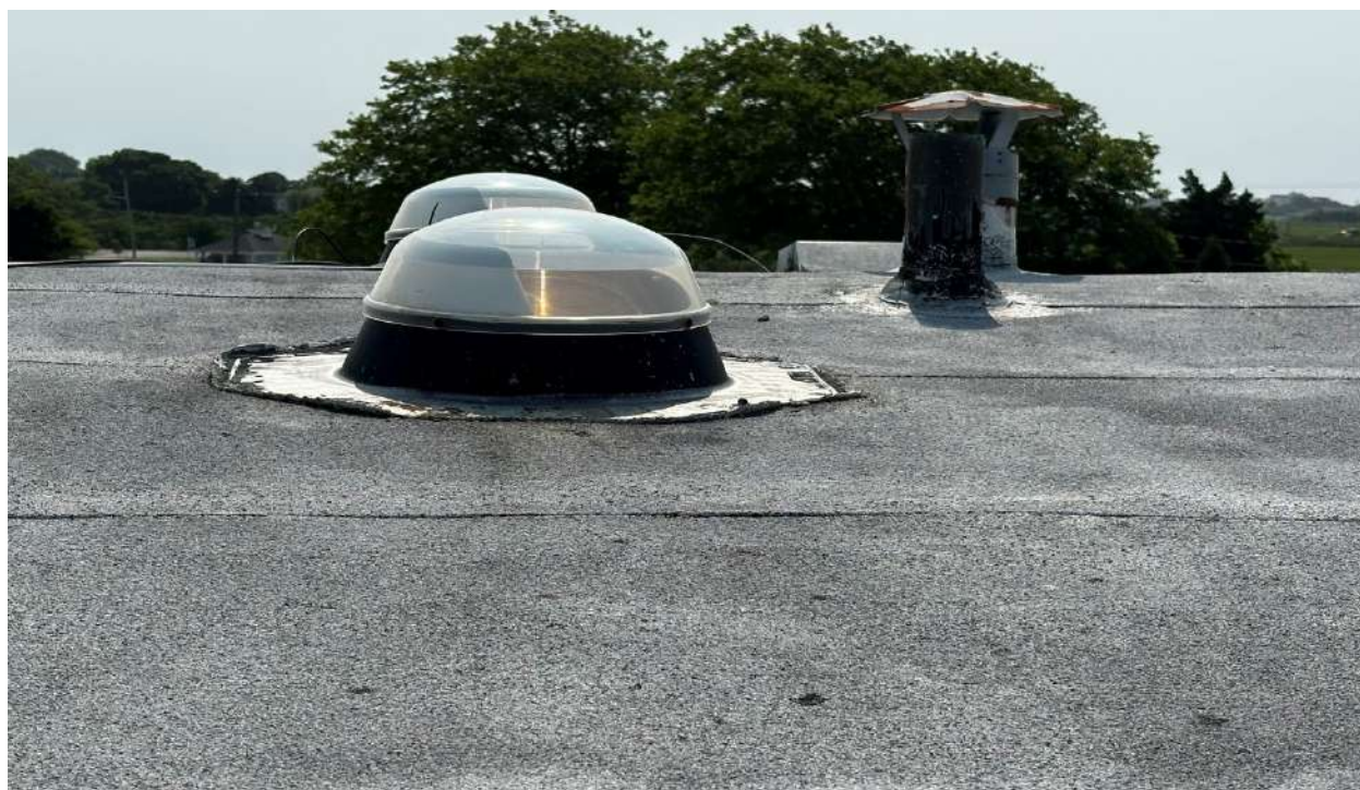
P-74 Solar Tube Skylight Un-flashed
