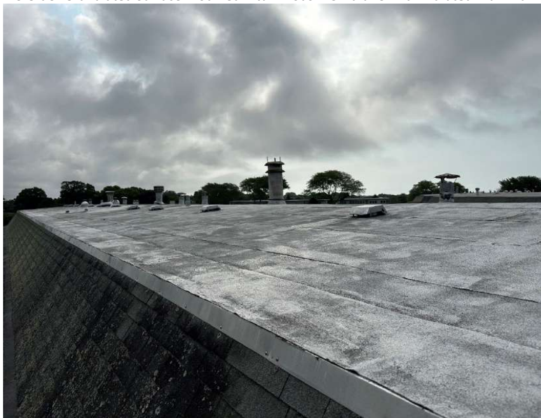
P-3 Older Granulated Surface Modified Bituminous Membrane With Fibrated Aluminum Coating
