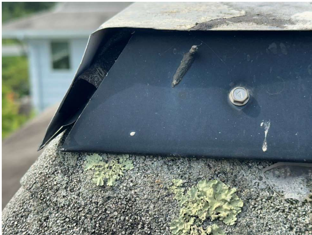
P-43 Delaminating Shingle
