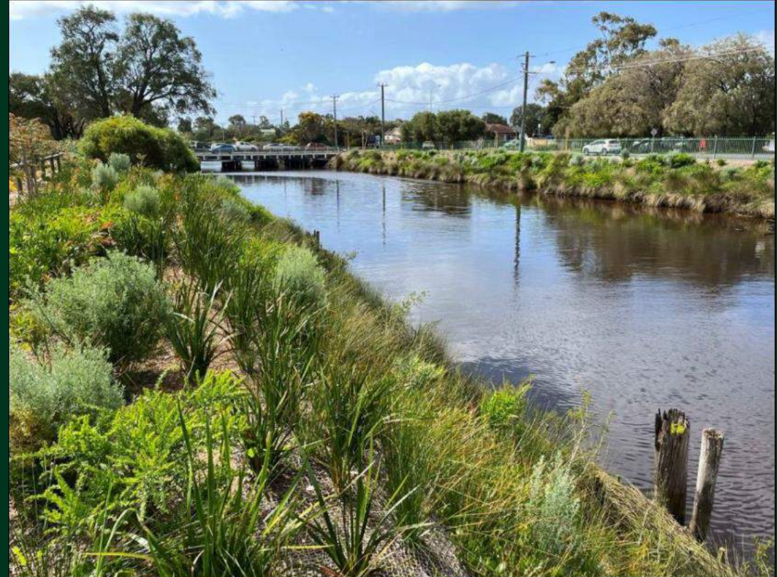
Image credit: A. Johnston, Vasse Diversion Drain Busselton AFTER
