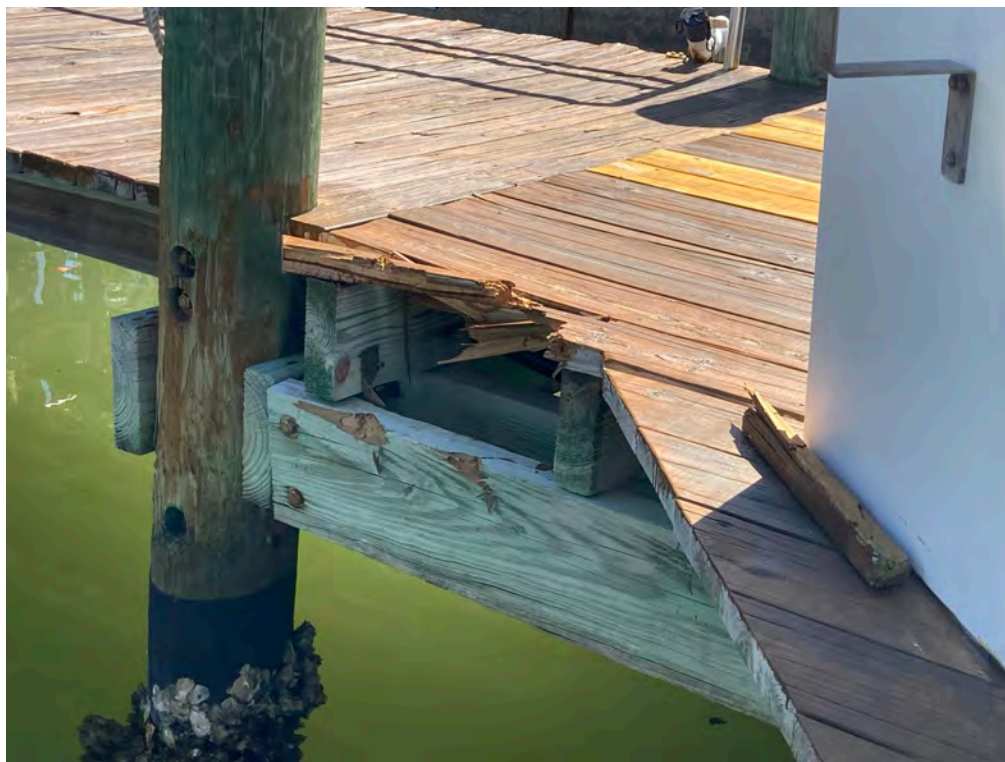
Figure 22: Broken Deck Board
