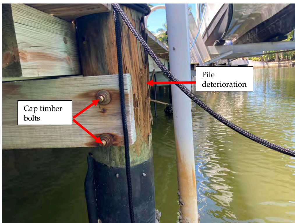
Figure 18: Close Up Pile Deterioration, Dock Framing
