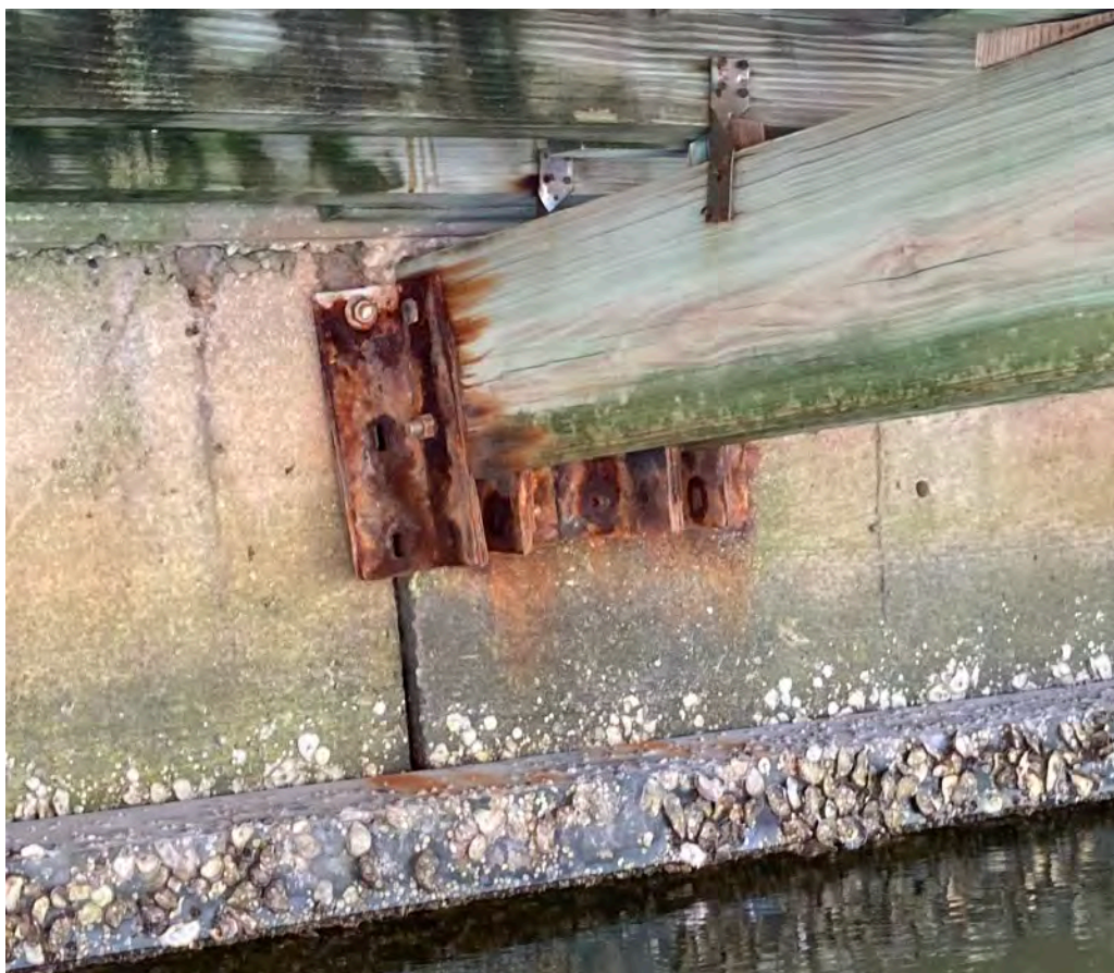
Figure 17: Hardware Connecting Fixed Dock to Seawall Panel
