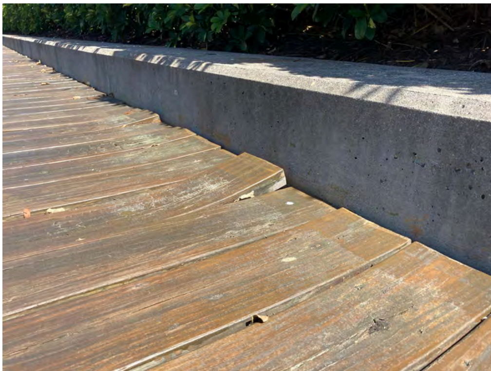
Figure 20: Warped Deck Boards
