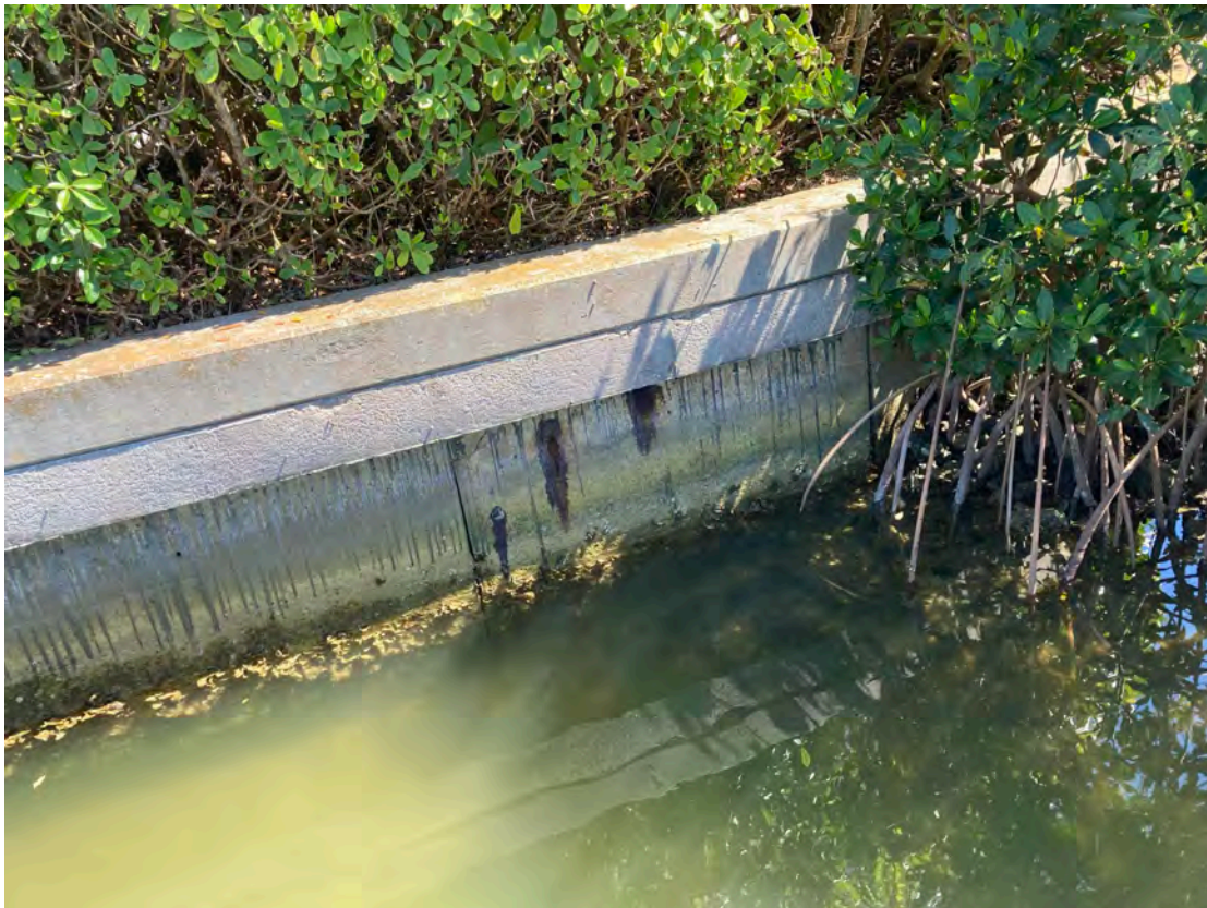
Figure 11: Minor Rust Bleeding (seen in 2017 report as well)
