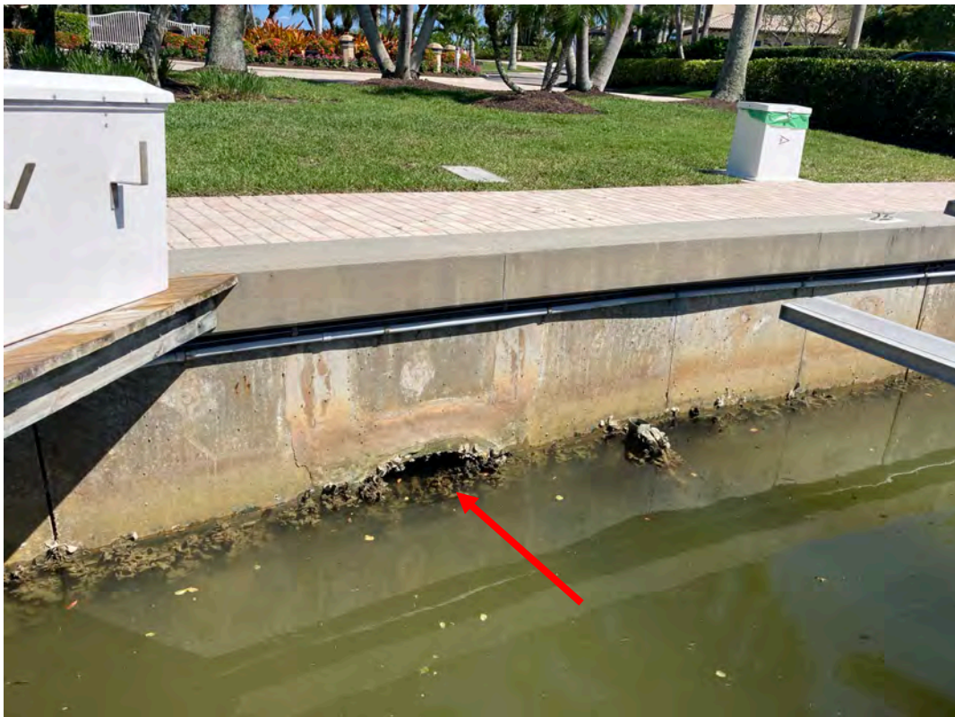
Figure 8: Stormwater Pipe Inside Basin
