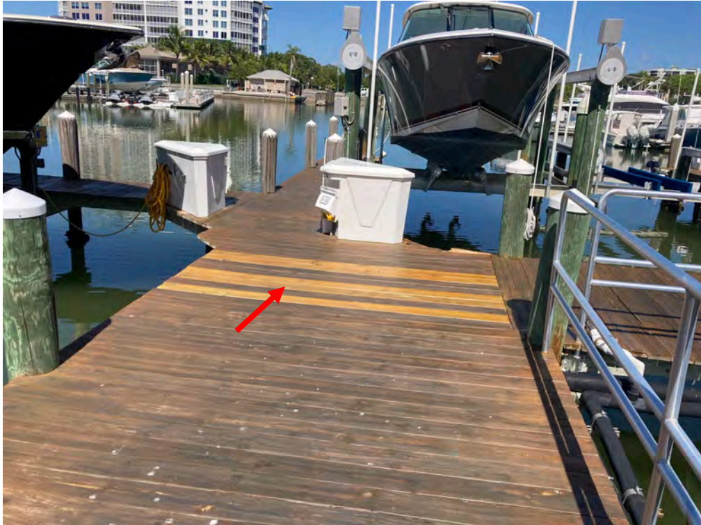
Figure 21: Recently Replaced Deck Boards
