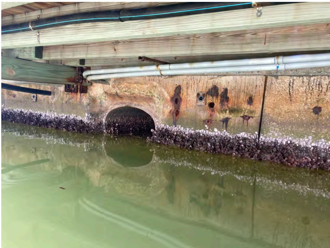
Figure 13: Stormwater Pipe, Panel Crack, Rust Bleeding (seen in 2017 report)
