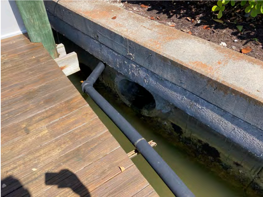
Figure 12: Stormwater Pipe
