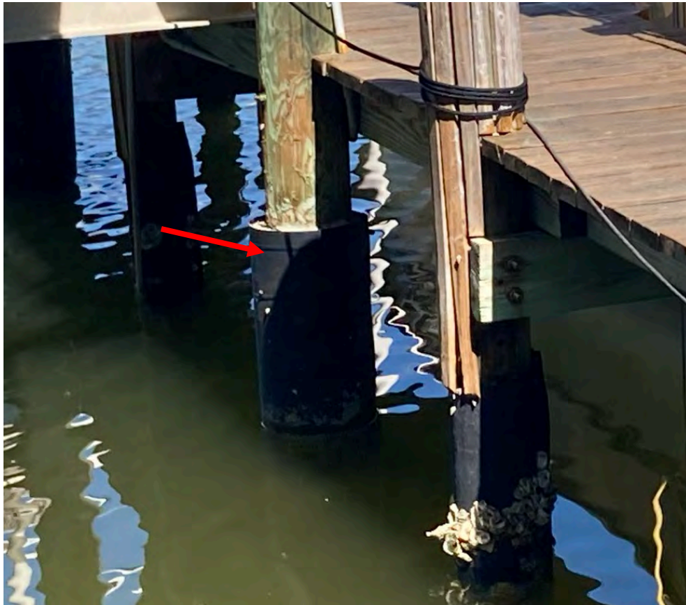
Figure 23: Pile Repair (concrete poured inside sleeve around the pile)
