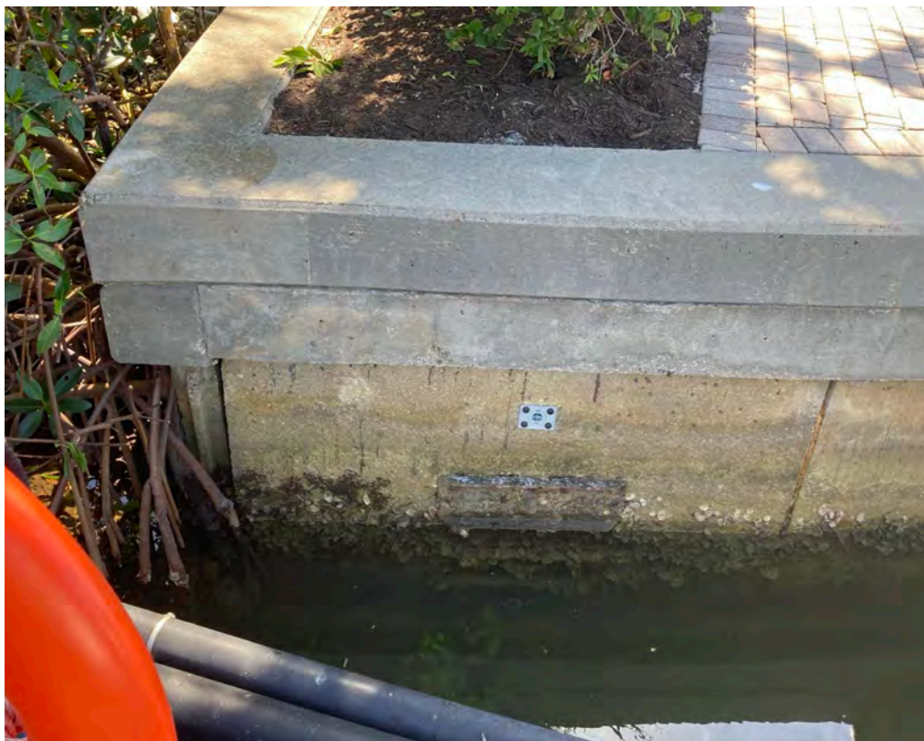
Figure 14: Seawall C East Termination, Helical Tieback Channel and Weephole
