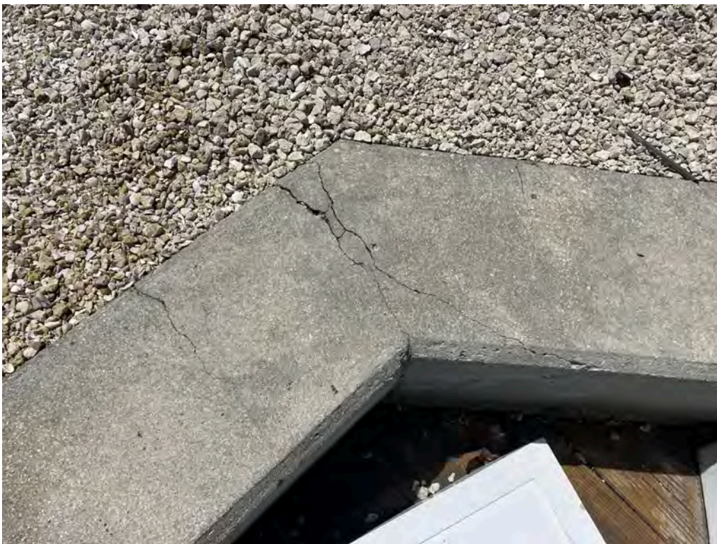
Figure 5: Seawall Cap Crack at Directional Change
