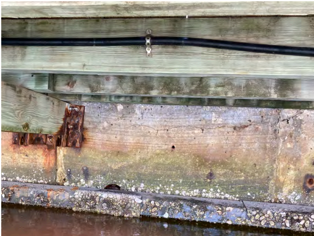
Figure 4: Horizontal Seawall Panel Crack
