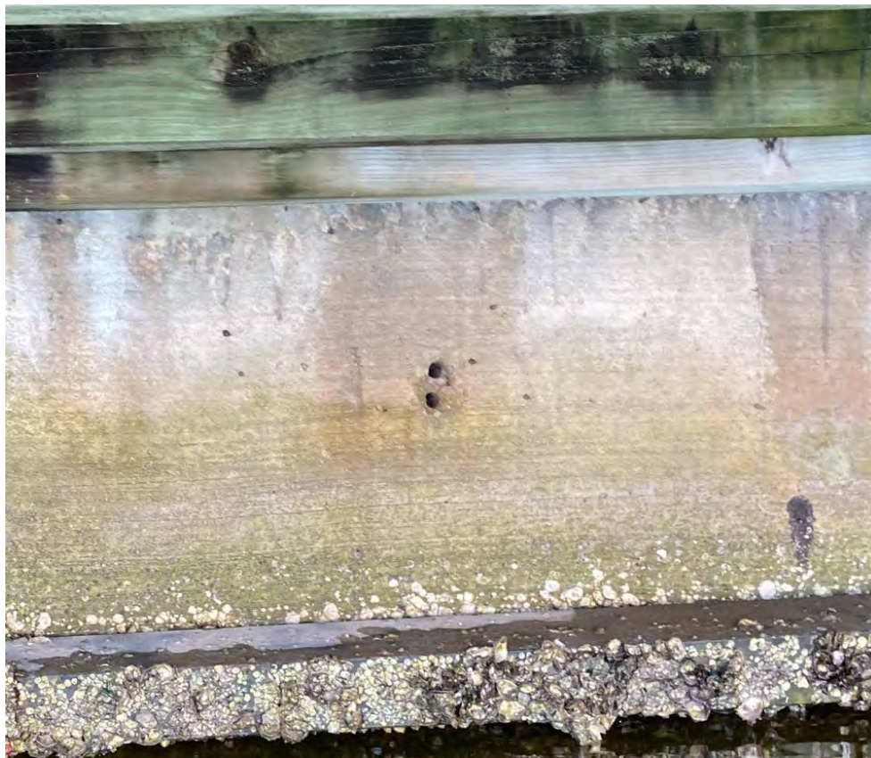
Figure 3: Extra Weepole Drilled
