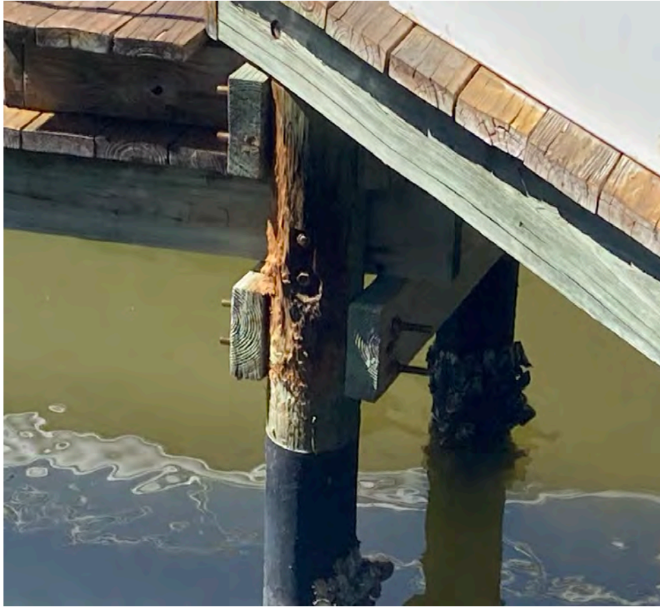
Figure 25: Severely Deteriorated Dock Pile
