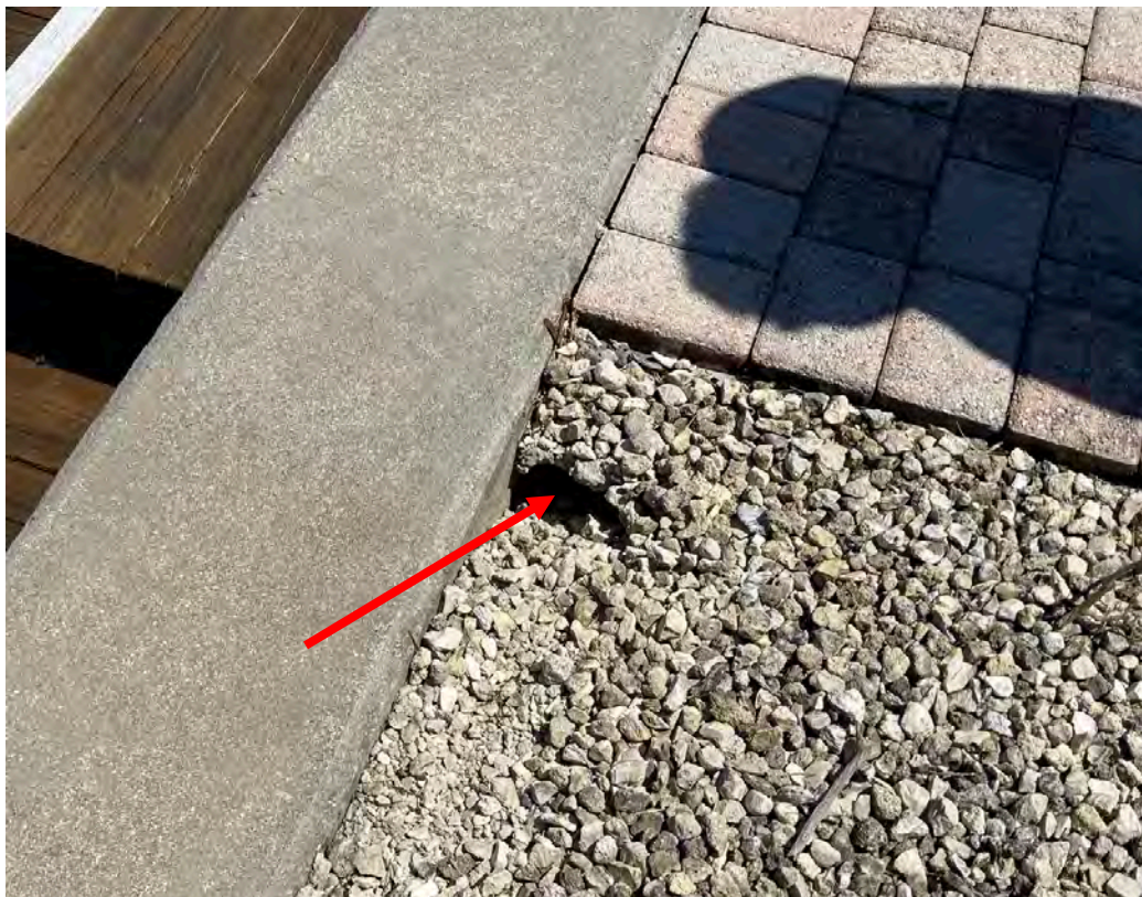
Figure 7: Minor Loss of Backfill Behind Cap
