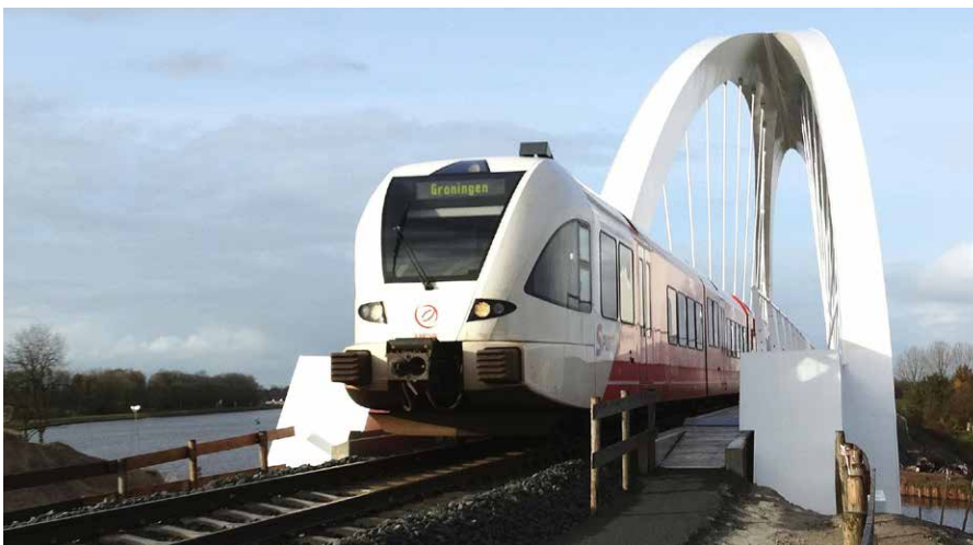
Fig 8 -- The completed Bert Swart Bridge across the Van Starckenborgh Canal in Zuidhorn, the Netherlands, handles two passenger trains per hour on weekdays, as well as freight traffic as needed. The 200-meter long 1,700-ton steel bridge blends architectural beauty and strength. The Xypex-coated concrete rail bed will lower mainenance costs and extend the life of the bridge.
