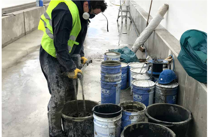
Fig 5 -- Totech of the Netherlands is the distributor of Xypex products for Belgium, the Netherlands, and Luxembourg (Benelux). Here, a worker mixes a batch of Xypex Concentrate for application to the bridge deck.
