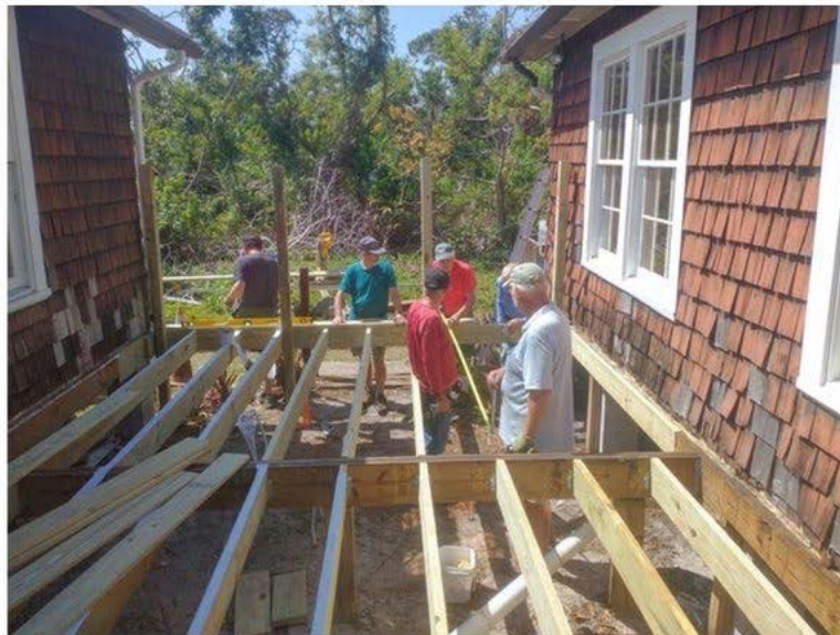
Tear Out and Structural Start of the Price House Middle Deck
