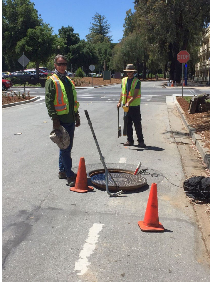
Galen Schmidt and Rob Donzanti marking utilities for a manhole relocation project along Panama Street.
